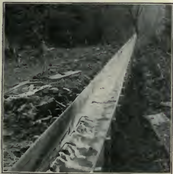
A Well-Built Sluice.
