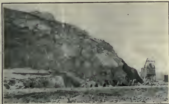
Fig. 5. Before Firing Blast.
