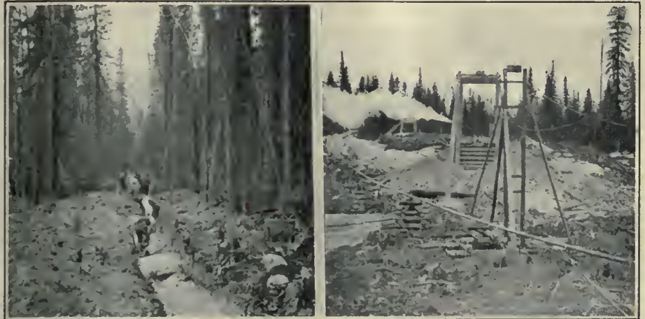
TRENCHING TO PROSPECT VEINS ON LOW GROUND.
