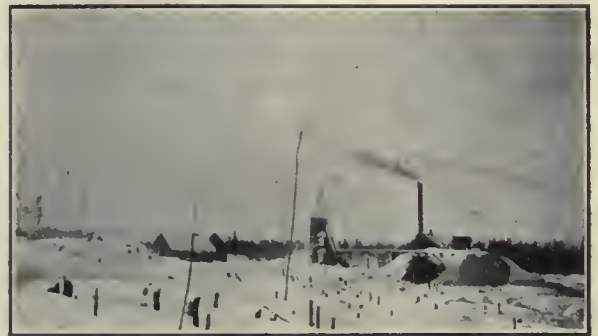
Hollinger Mine. Shaft No. 1, Stock Pile, and Test Mill.
