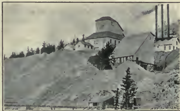
Logan Shaft, Stratton's Estate Co., Cripple Creek.
