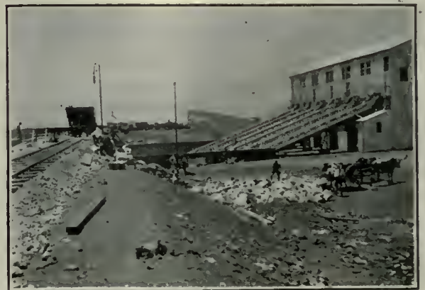
Gold-Recovery House. Randfontein Central.
