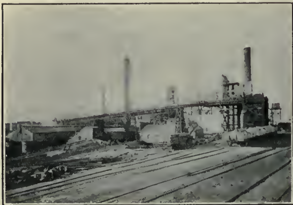
Main Shaft, Broken Hill Proprietary.
