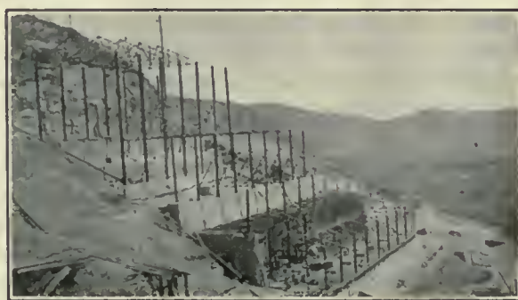
La Blanca Mill, Foundation and Framework.
