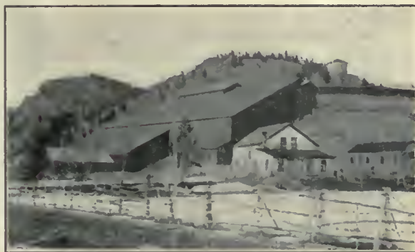
North Homestake Mill, Maitland, South Dakota.
