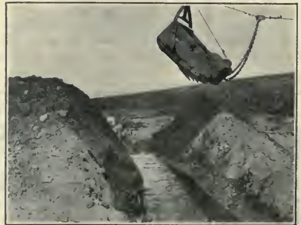
Dumping the Bucket.
