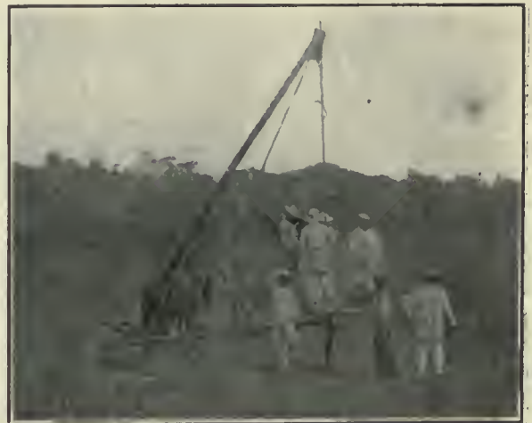
Drilling With Spring Pole.
