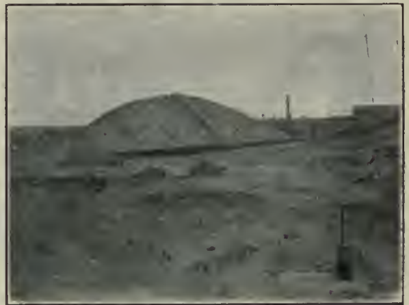
VACUUM PLANT REMOVING OROYA-EXPLORATION DUMP FOR RE-TREATMENT.
