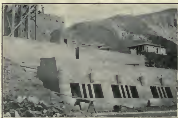
Stamp Foundations and Ore-Bins, Nevada Hills Mine.
