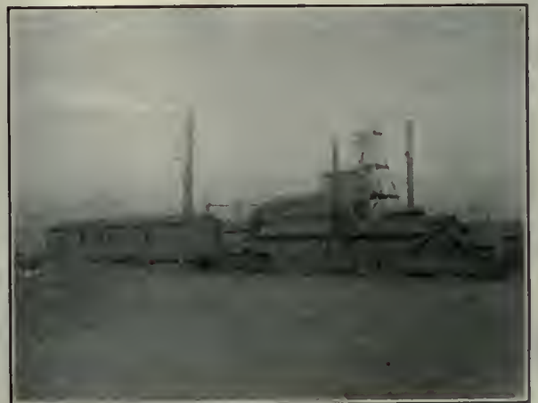
FIG. 2. STACK OF ROASTING PLANT, GIVING OFF ARSENIOUS OXIDE FUME.
