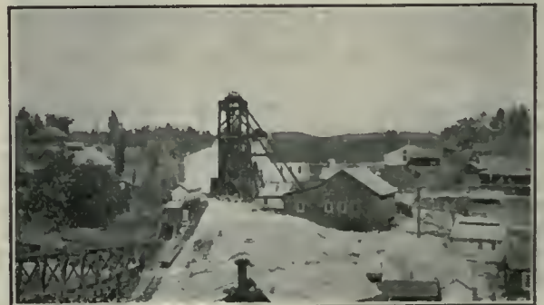
NEW SHAFT, LIGHTNER MINE.
