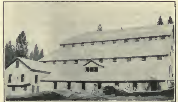
Cyanidation Plant, Empire Mines.
