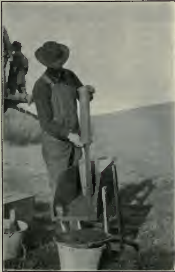
Emptying the Drilling Pump.
