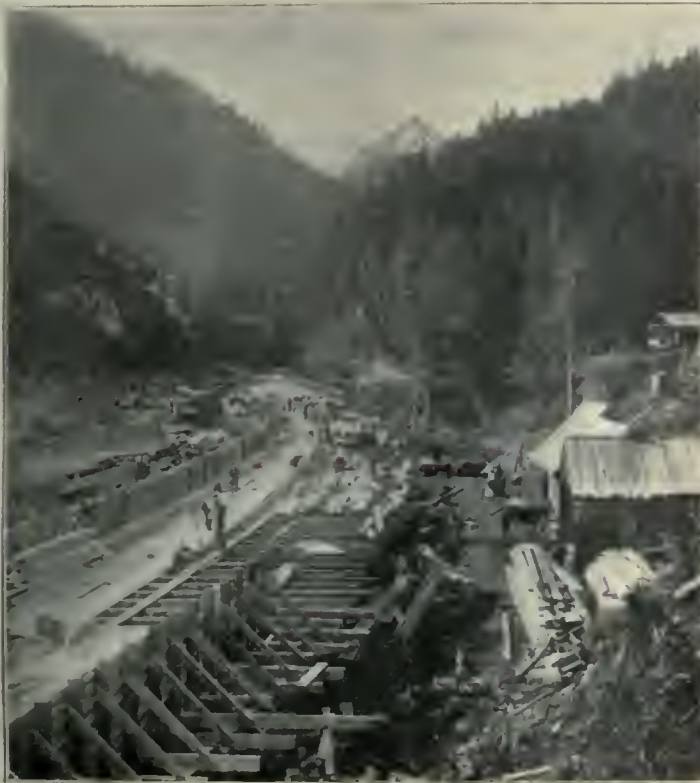
Main Flume, Porcupine Mine.
