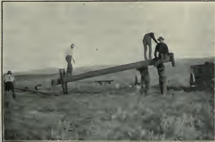
Pulling the Pipe.
