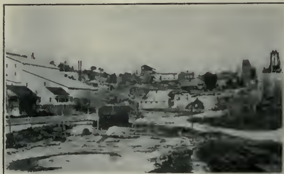
LIGHTNER MILL AND MINE, ANGELS CAMP, CALIFORNIA.
