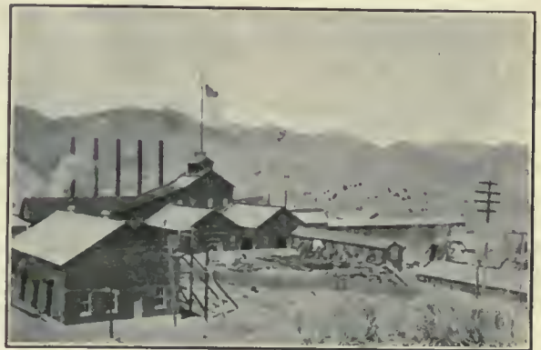
C. & C. Shaft With Sub-Station of Gen. Elec. Co. in Left Foreground, Virginia City, Nevada.
