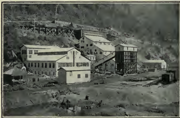
HERCULES MILL AND SLIME-PLANT, WALLACE, IDAHO.
