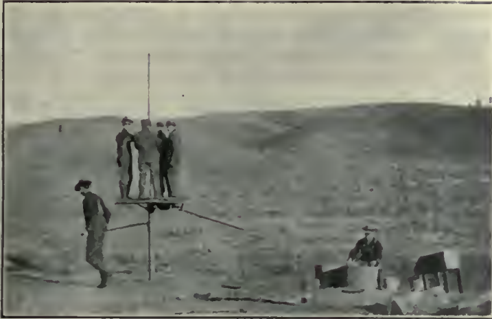
Set-up of Drill and Rotation by Hand.
