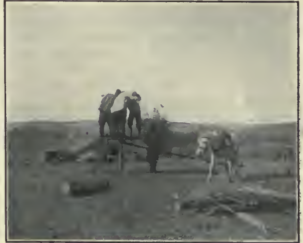
Drilling Frozen Ground. Notice Tank for Heating Water.
