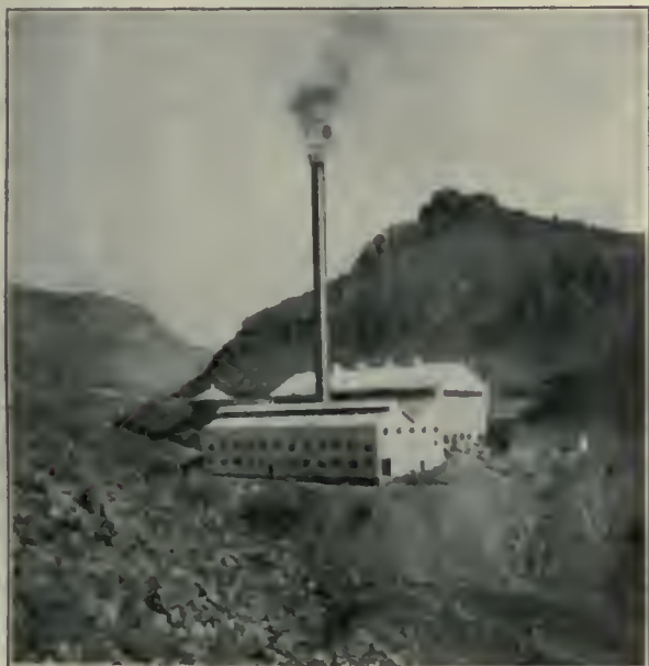
Copper Queen Power Plant.
