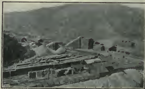
Bunker Hill & Sullivan New Mill.
