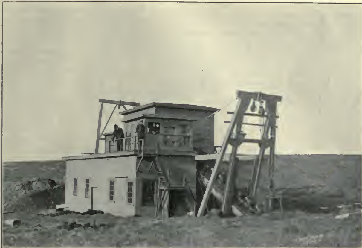
Arctic Gold Dredging Co.'s Dredge, Saunders Creek, Nome District. (Built by Union Iron Works.)
