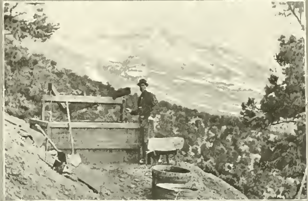
A HAND-JIG WORKING ON TUNGSTEN ORE.
