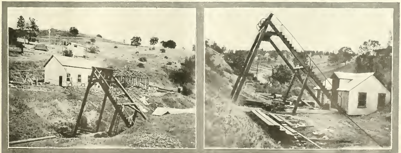
RE-OPENING OF THE EUREKA MAIN SHAFT, SHOWING TEMPORARY HEAD-FRAME.
