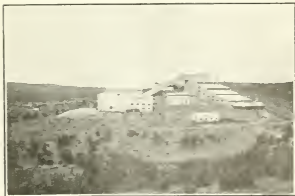
NEW MILL OF THE BURRO MOUNTAIN COPPER CO., TYRONE, NEW MEXICO.
