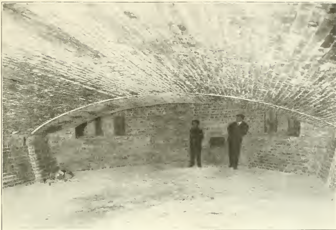
FIG. 5. FRONT END OF NO. 6 REVERBERATORY FURNACE. THE INDEPENDENT VERB ARCH IS SHOWN, SEPARATED BY A 4-INCH JOINT FROM THE REST OF THE ROOF. THIS JOINT CLOSES BY EXPANSION WHEN THE FURNACE IS HOT. BETWEEN THE MEN IS THE SLAG-HOLE OR SKIMMING-HOLE.
