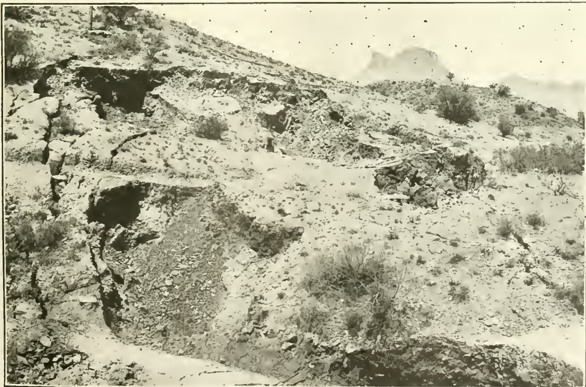
CAVING OF THE SURFACE AT RAY, ARIZONA.
