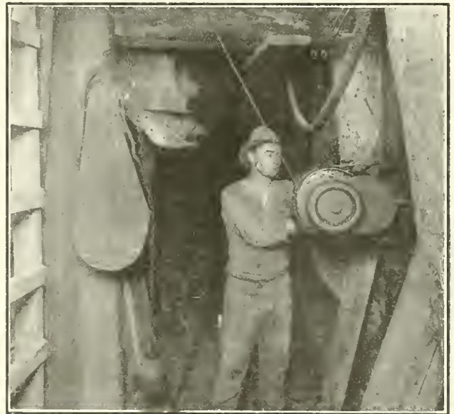
THE LEADVILLE DRILL-COLUMN HOIST IN USE.
