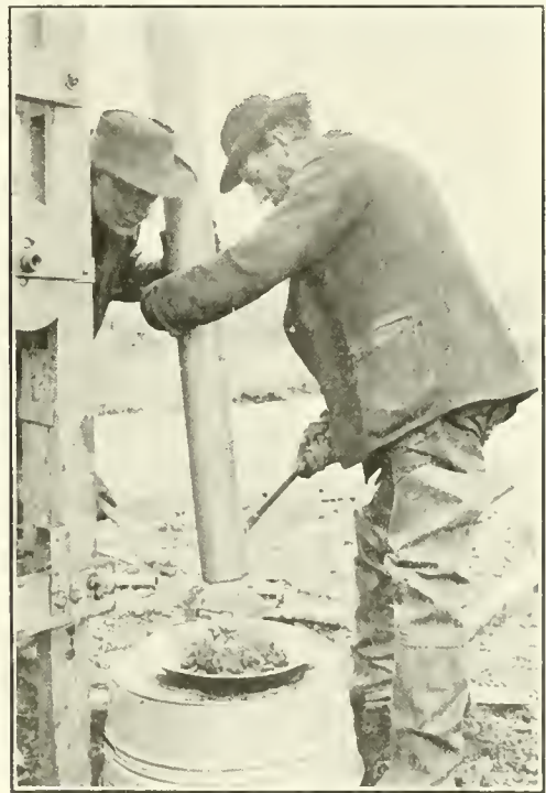
REMOVING THE CORE.
