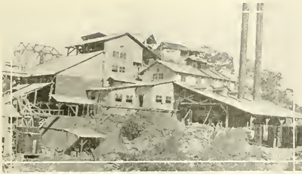
THE CYANIDE PLANT.
