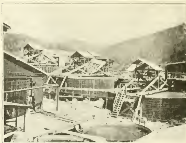
CYANIDE PLANT, MELONES MINE, CALAVERAS COUNTY, CALIFORNIA.
