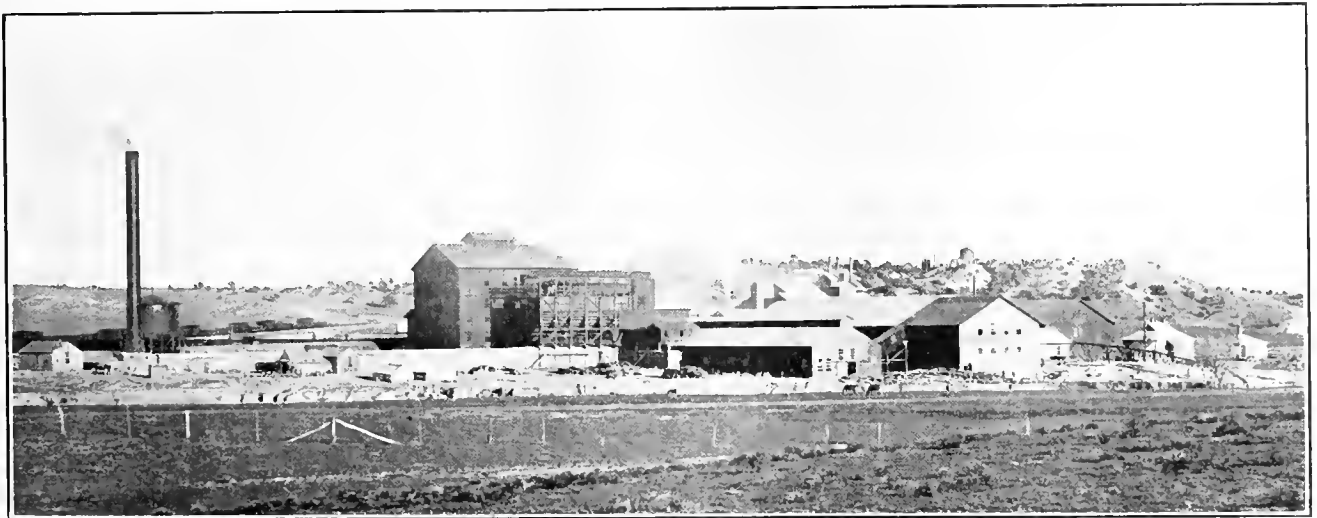
THE METALLIC WORKS AT FLORENCE, COLORADO, 1896.
