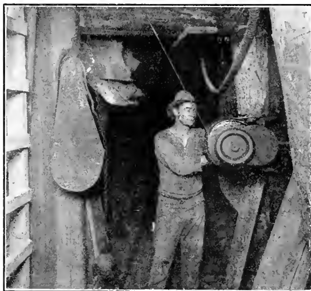
THE LEADVILLE DRILL-COLUMN HOIST IN USE.
