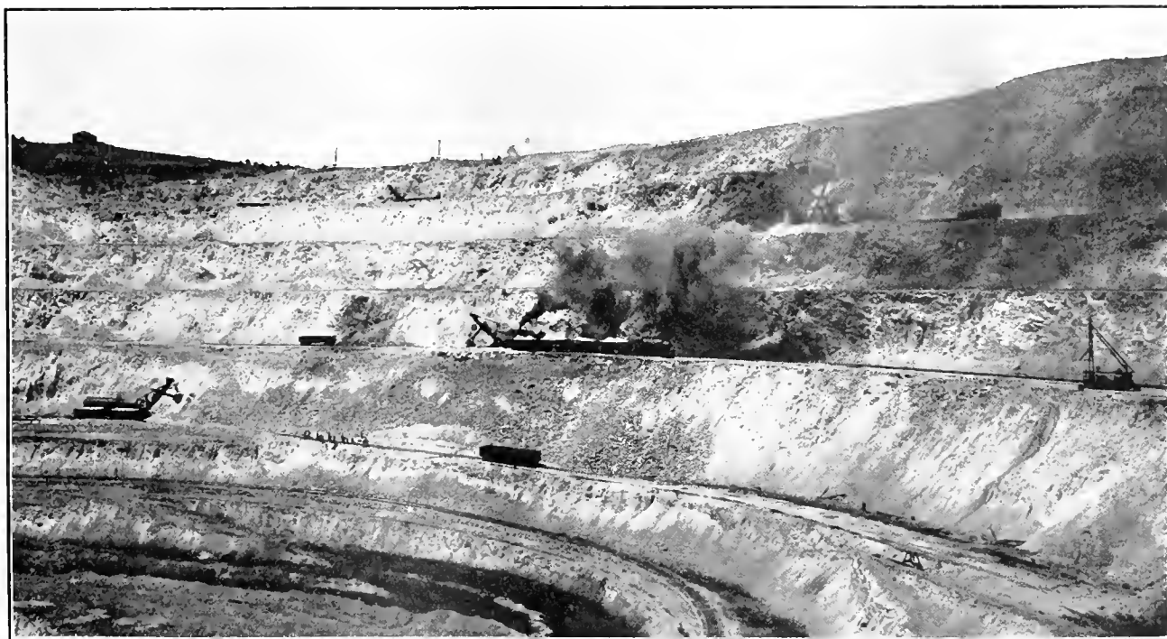
WHERE 'WELL-DRILLERS' ARE USED TO DRILL HOLES FOR BLASTING. THE PIT OF THE NEVADA CONSOLIDATED COPPER CO., ELY.
