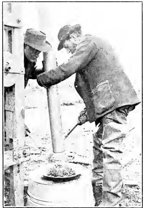
REMOVING THE CORE.
