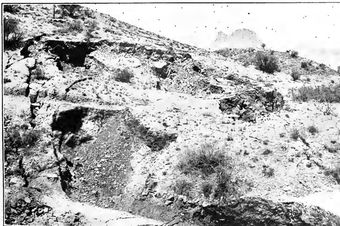
CAVING OF THE SURFACE AT RAY, ARIZONA.
