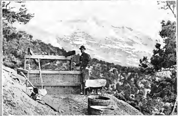
A HAND-JIG WORKING ON TUNGSTEN ORE.
