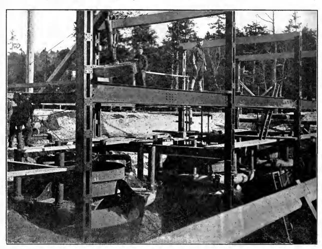
Steel Structure in fore-bay supporting the three compressor-heads over each shaft. On the head-piece to the left a space is open wherein the pipe-head containing the small air-inlet tubes hanging on the derrick, just above, is to be placed.
