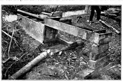
Delivery Vat. First Settling Vat, and Sand-Pump.
