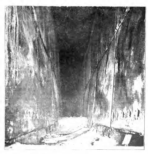
Interior of Blast Furnace at Hearth-Level.
