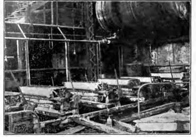
Zinc-Dust Precipitation at the Mercur Mill, Utah. Agitation Tank in the Background and Filter-Presses in Front. Compressed-Air Receiver to the Right.
