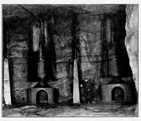
Fig. 5. Flash-light view of the three steel tubes, which extend through roof of air-separating chamber and are connected in lower end of compressor shaft. The photograph also shows the division wall between the tubes, placed there to prevent the water of one compressor from interfering with the other.
