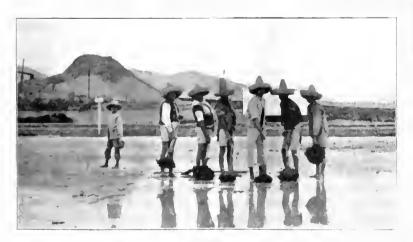
Sweeping the Mercury and Amalgam tnto the Sump; the Last of the Charge on the Patio.
