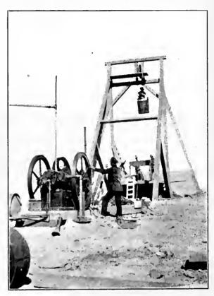
Original Combination Shaft, Man in Bucket. (Site Now Occupied by Large Open-Cut.)
