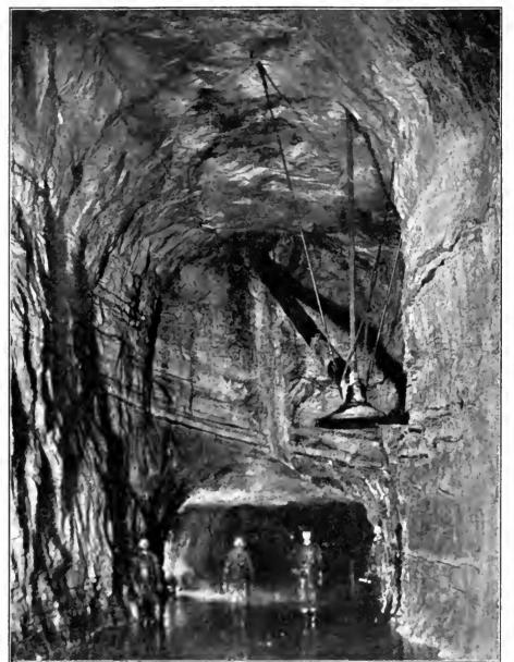
Fig. 2. Flash-light view showing outlet end of air-separating chambers. In the upper corner the end of the 24-in. air-main is shown with a strainer at its end; leading down with a saucer piece on its end is the 12-in. blow-off pipe. The low tunnel at the bottom is the water escape which connects with a tail-race shaft.
