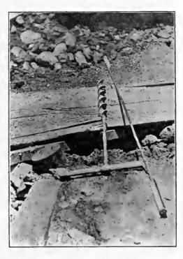
Fig. 3. Auger and Gun for Block-holing.
