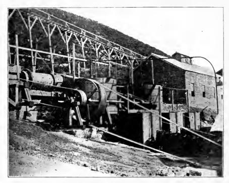
Tube-Mill and Experimental Cyanide Plant.
