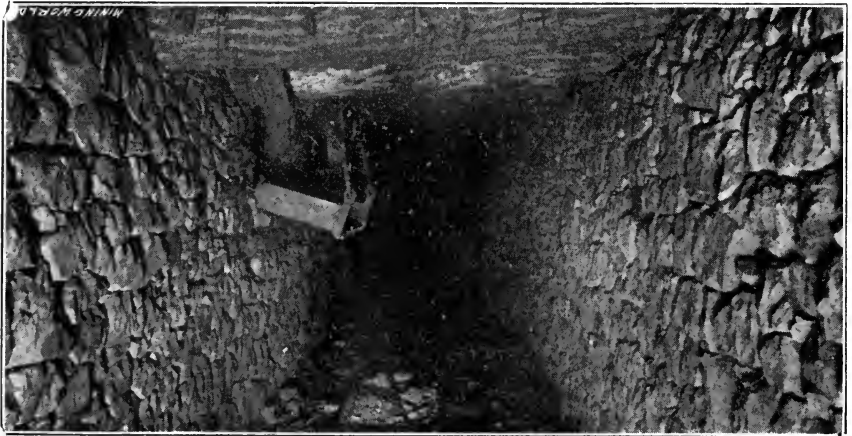
FIG. 55.—Dry-walled tunnel, Champion mine.
