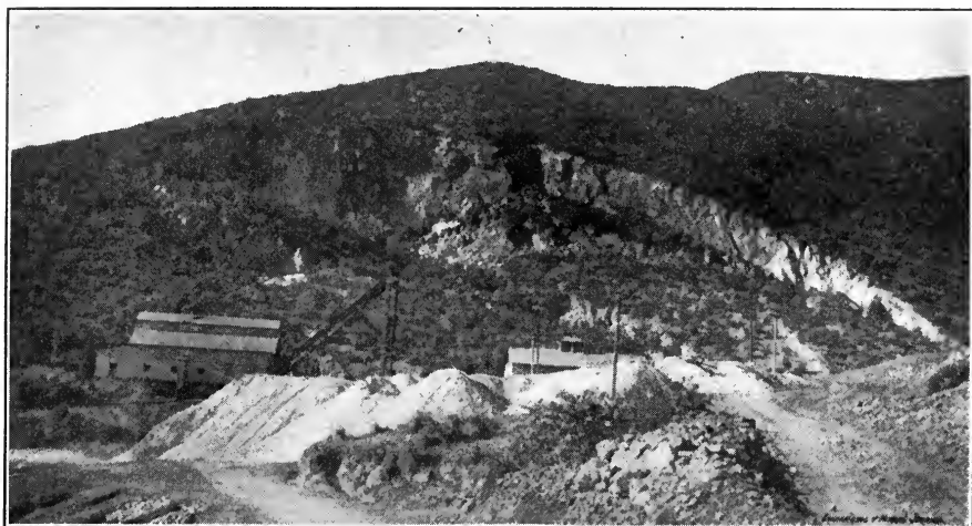
FIG. 103.—Caved ground, Veta Grande mine.
