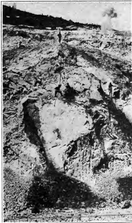
FIG. 31.—Trimming bank, Utah Copper mine.
