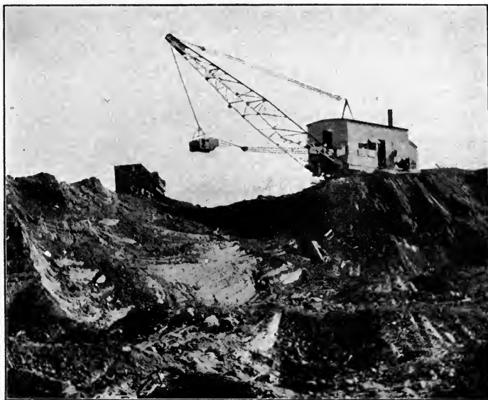
FIG. 25.—Drag-line excavator at Mayari, Cuba.
