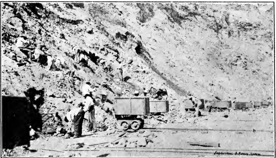
FIG. 35.—Openpit mining at Puertocitos.
