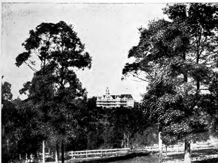
A sanitarium in the forest
