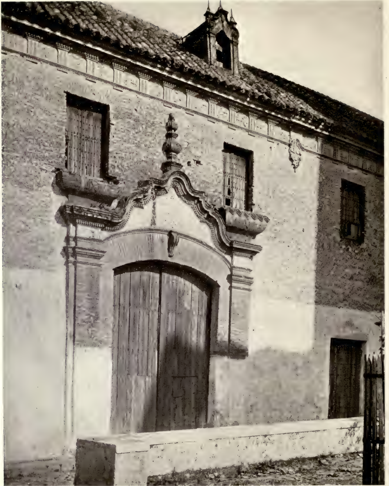
MARCHENA—A HOUSE ON THE CHURCH PLAZA
