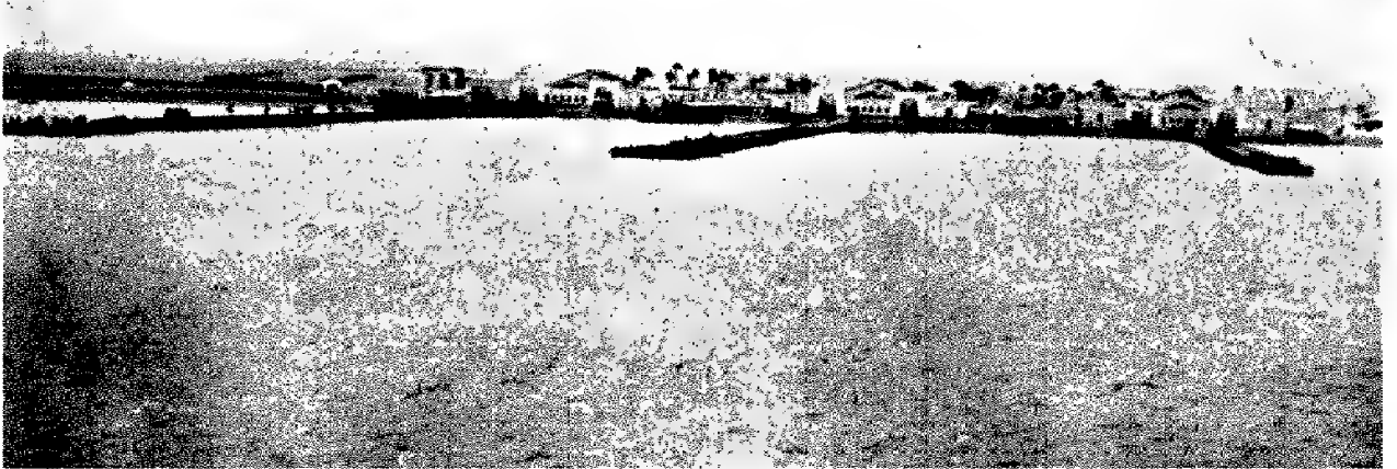
Tor Quarantine with its disinfecting machines & 3 quays
