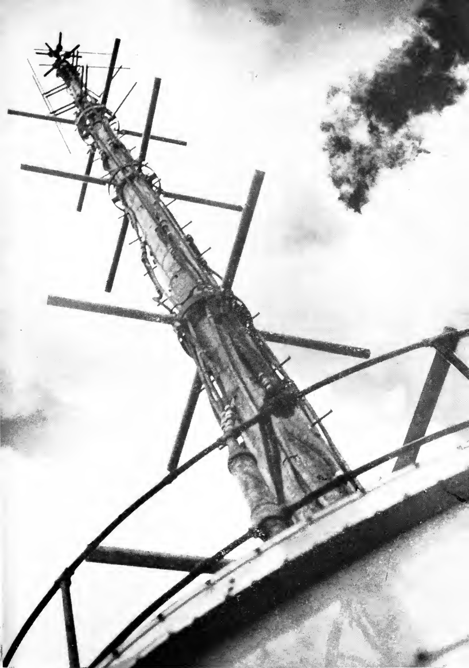
The highest man-made structure in the world, the NBC antenna atop the Empire State Building in New York City, greatly extends the area for transmission of television broadcasts.
