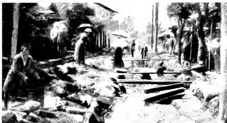
MAIN STREET AFTER THE FLOOD.
