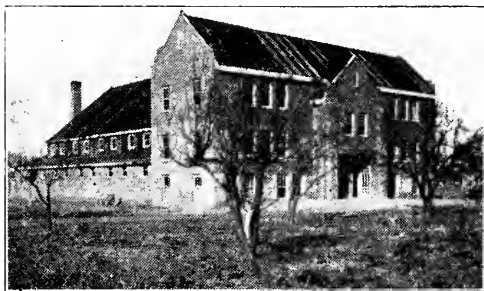
New Administration Building and Gymnasium
