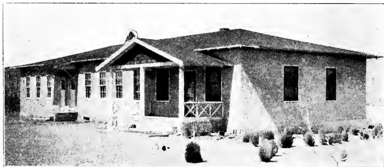
Alcalde Mission, Workers' Residence and School Building
