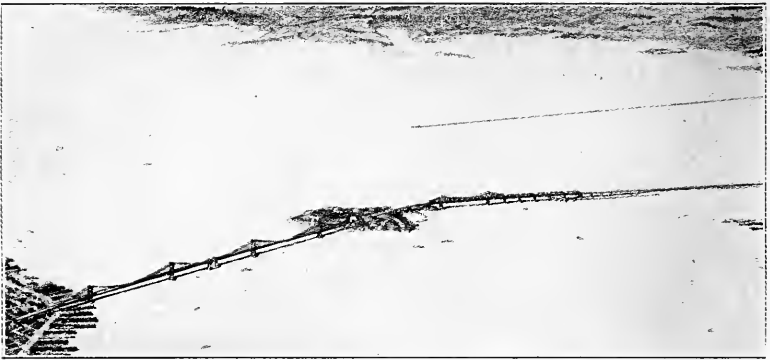
Famous San Francisco Bay Bridge Now Under Construction
