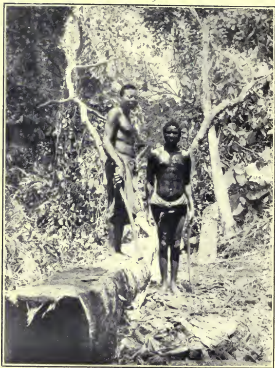
DRESSING TIMBER FOR BUILDING.
