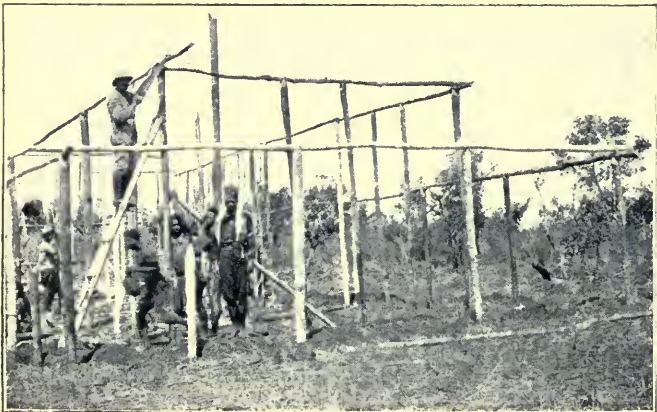
BUILDING A HOUSE AT DUNGU.
