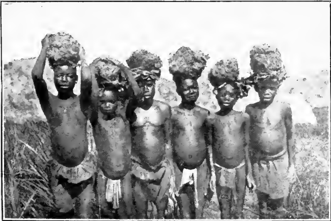
CARRYING MUD FOR HOUSE BUILDING.
