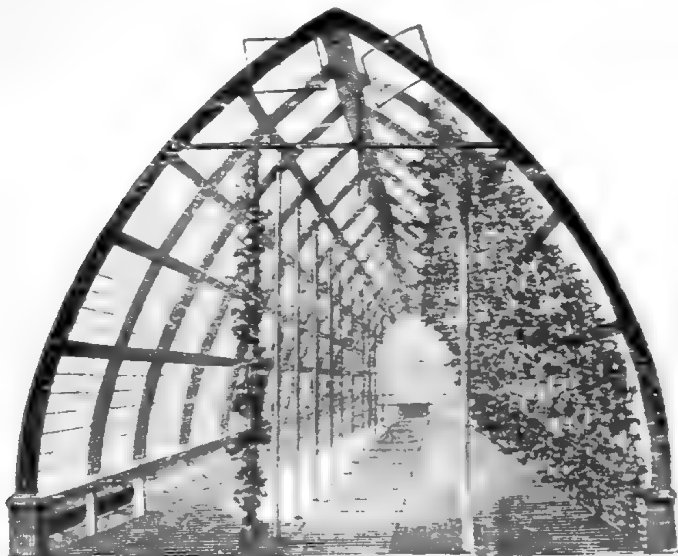
Inside view of the vine-grapeery of J. C. Green. Each station is 120 feet long.
