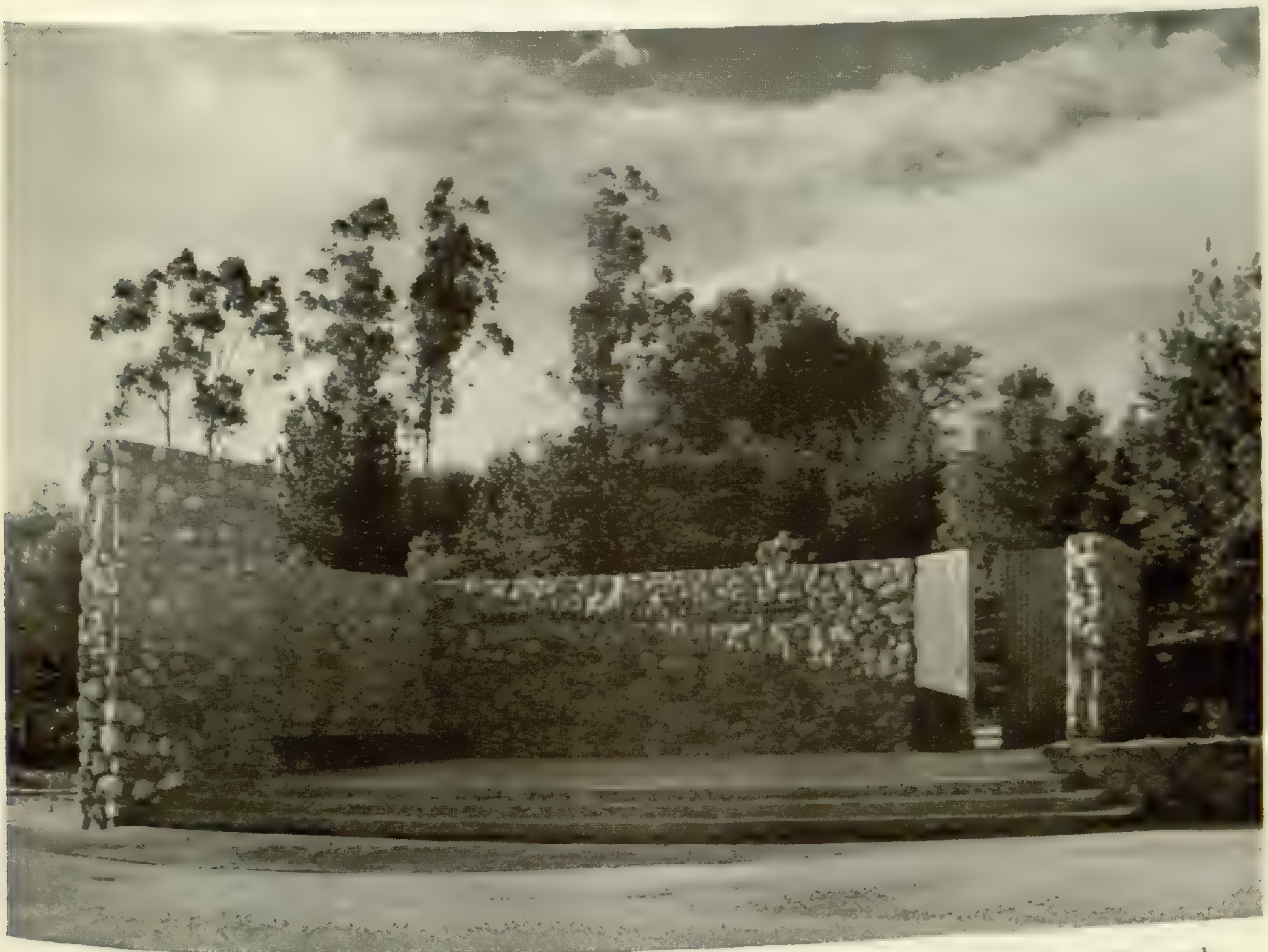
New main entrance gateway, constructed of native rock and redwood. Photo: Paul Kennedy
