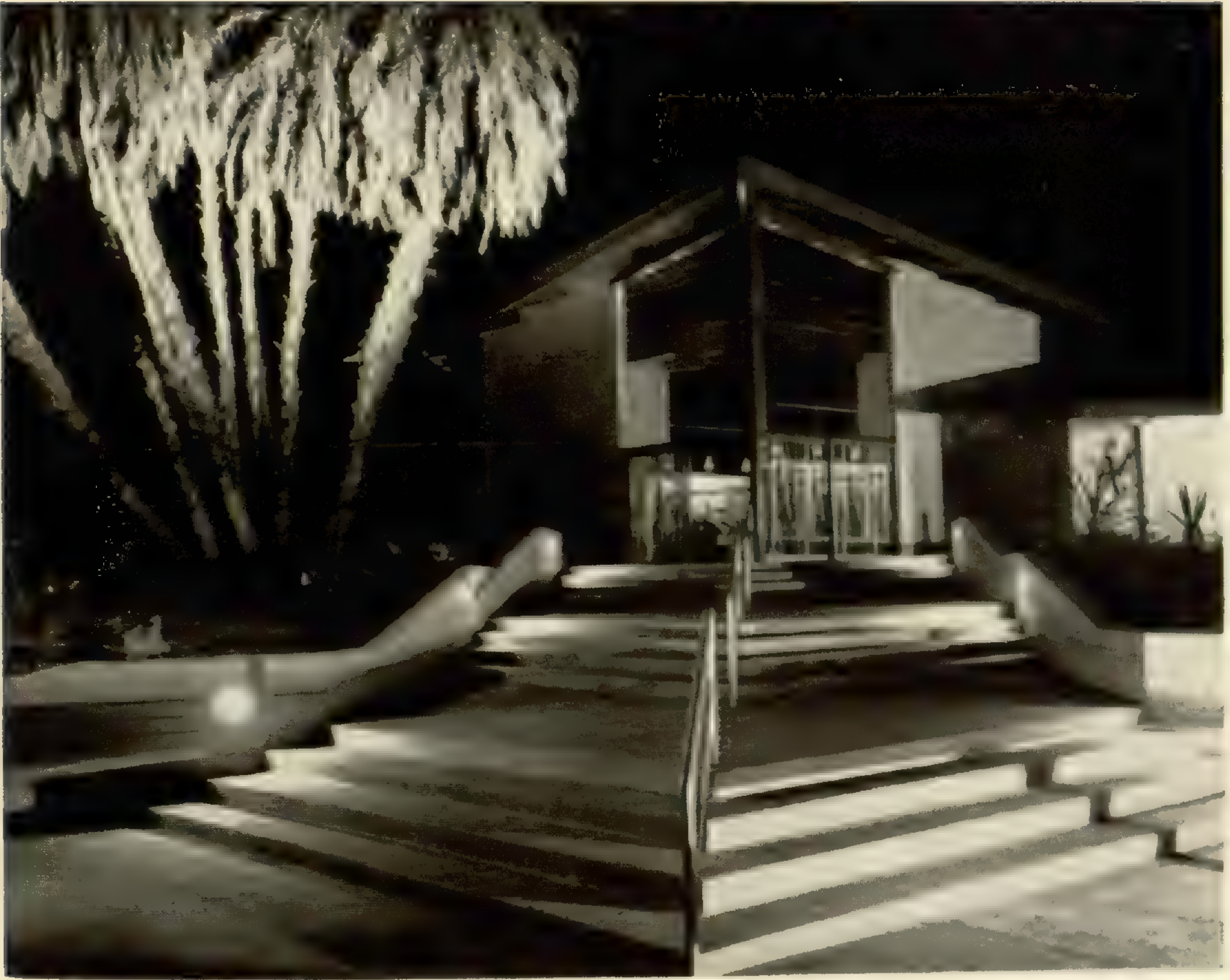
Night lighting of the Administration Building entrance creates interesting patterns of lights and shadows. Photo by L. B. Martin
