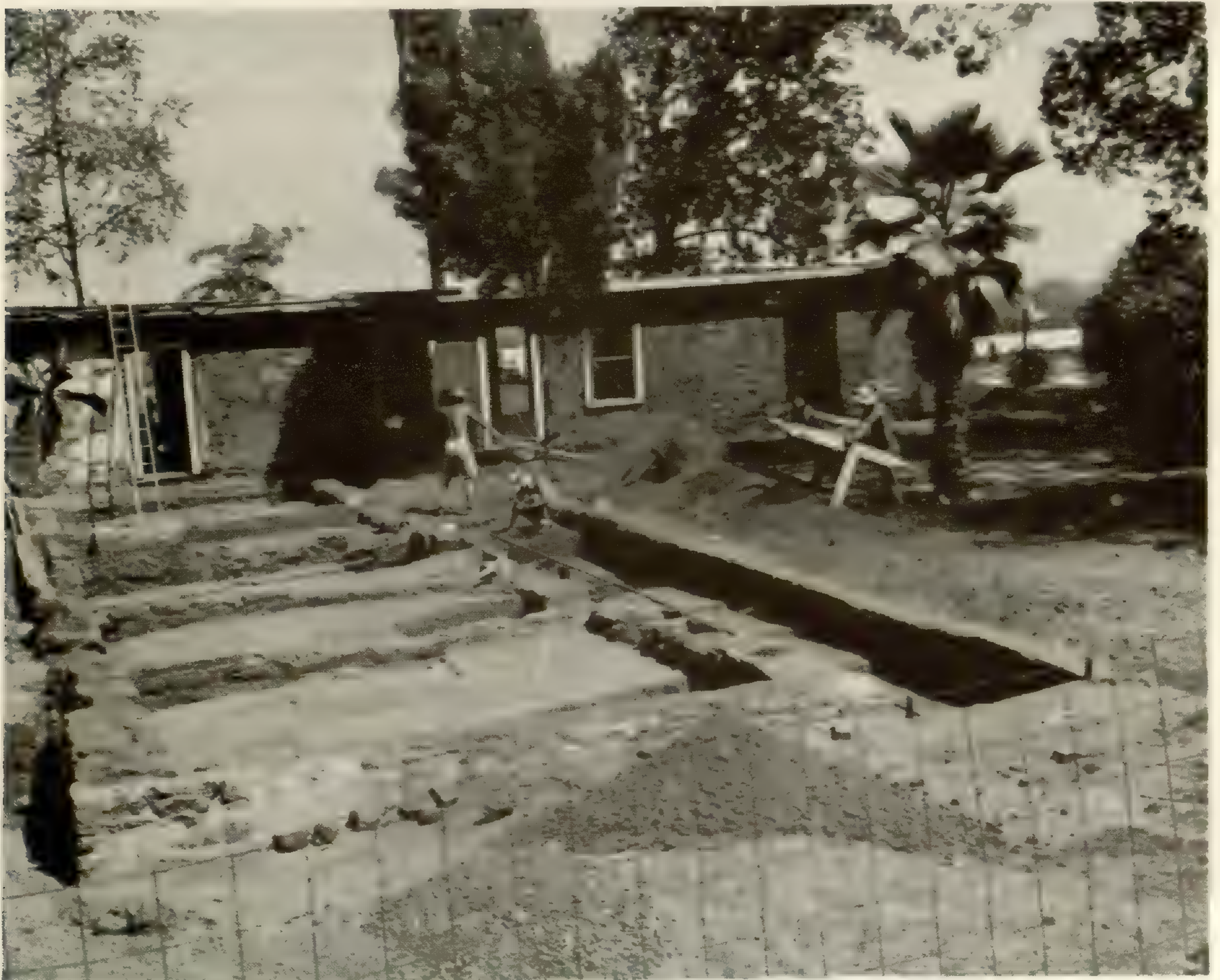
Hugo Reid Adobe and Foundation under Baldwin Annex. Looking east: Ken Dampf shovels out back dirt; Dr. Wallace cleans about pipe in pit; Gary Coon searches rocker screen.
