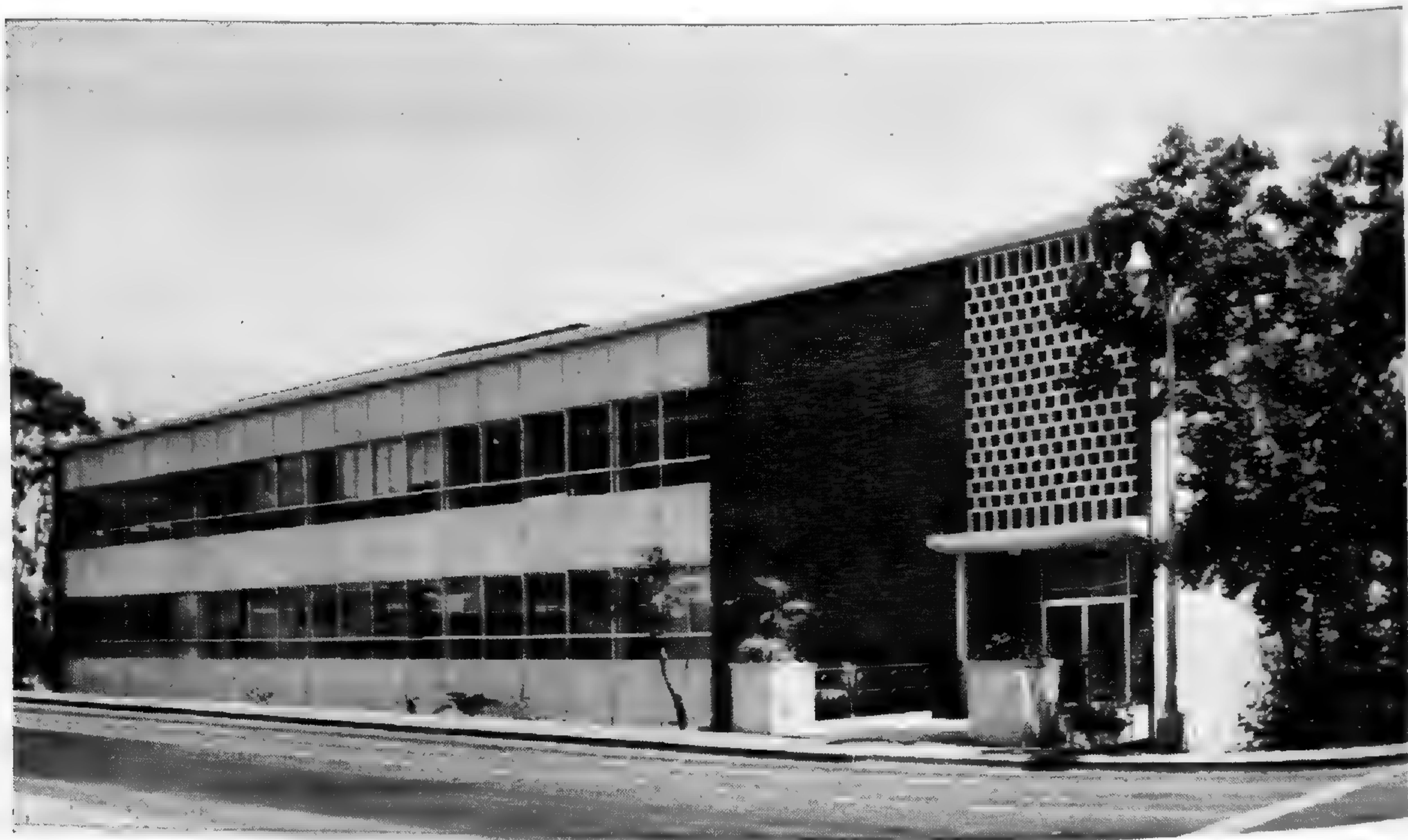
The new four-story (two levels are below this view) Botany Building at UCLA. Located between the Plant Physiology Building and the Botanical Garden, this newest facility rewards the student with an unusual opportunity to study botany in the closest proximity with the many necessary tools of this science.
