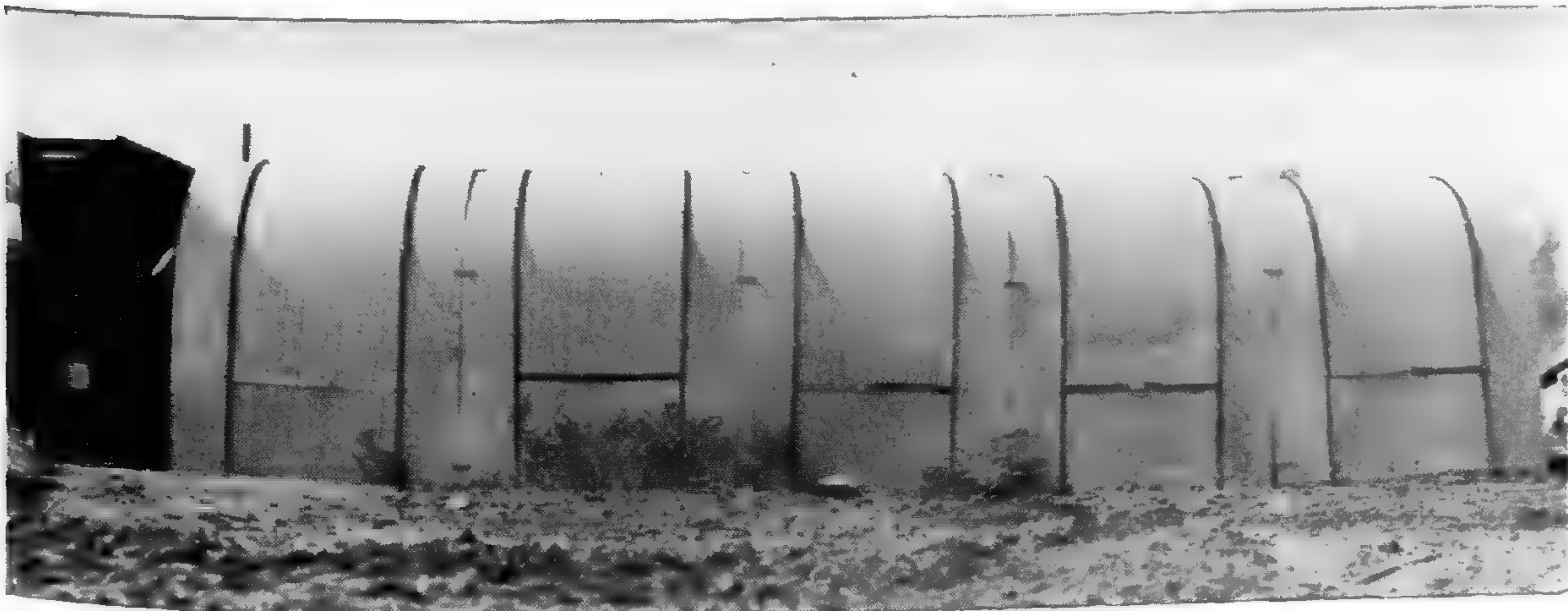
Figure 1. Second fire tunnel constructed of reinforcing steel and galvanized metal. Operational dimensions, 20' x 5' x 4'. Electric fan on extreme left.
