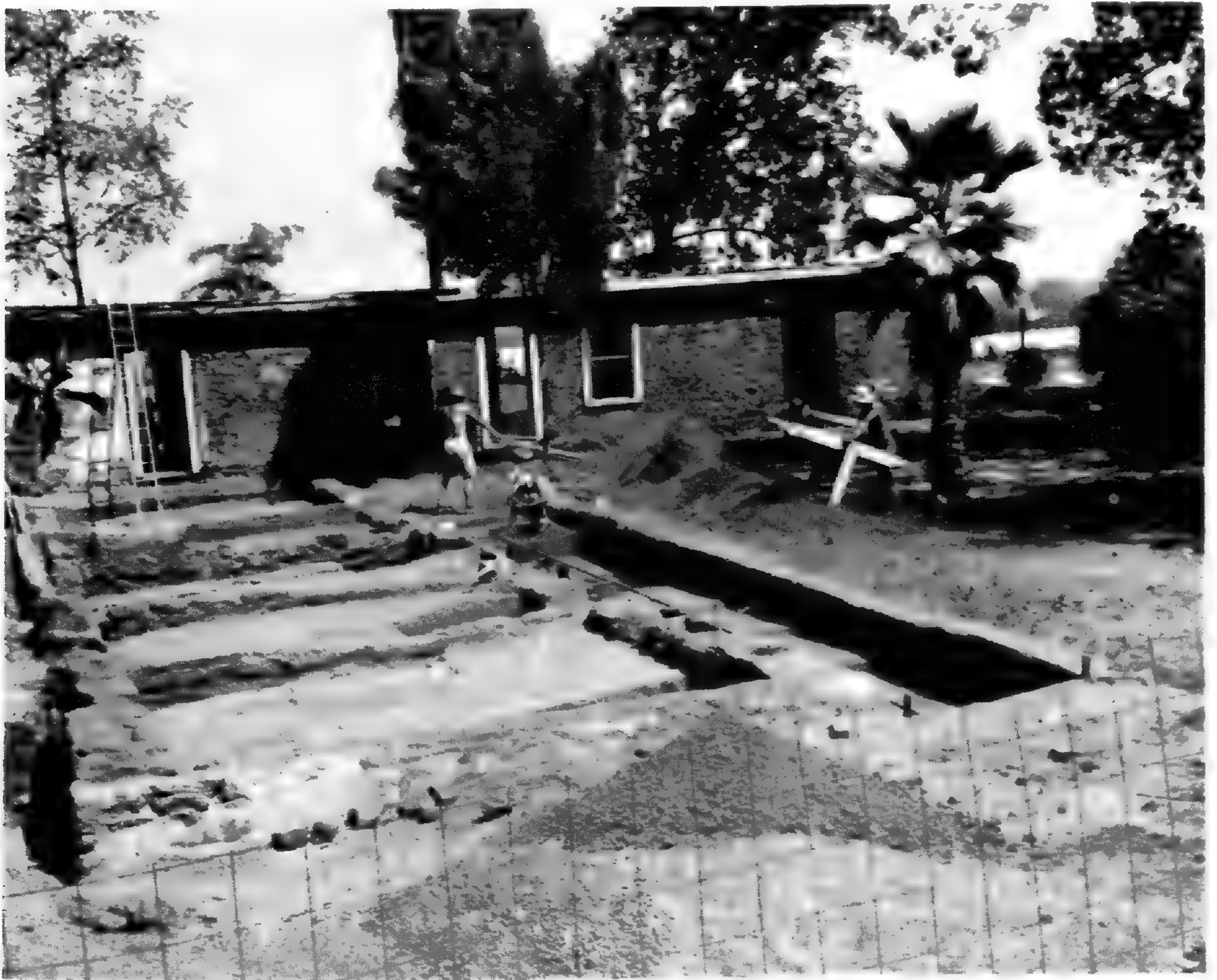
Hugo Reid Adobe and Foundation under Baldwin Annex. Looking east: Ken Dampf shovels out back dirt; Dr. Wallace cleans about pipe in pit; Gary Coon searches rocker screen
