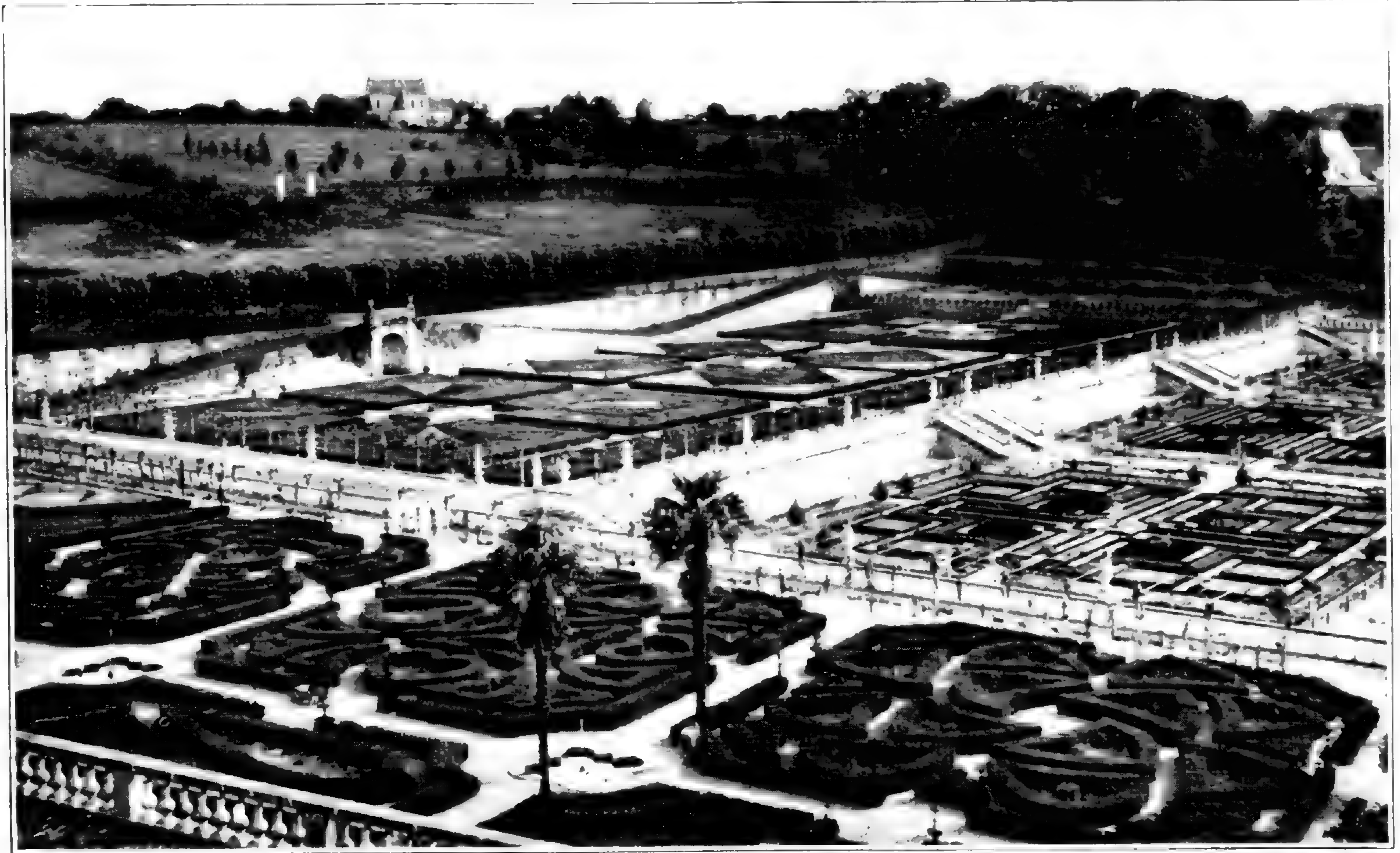
FORMAL GARDEN AT VILLANDRY.
