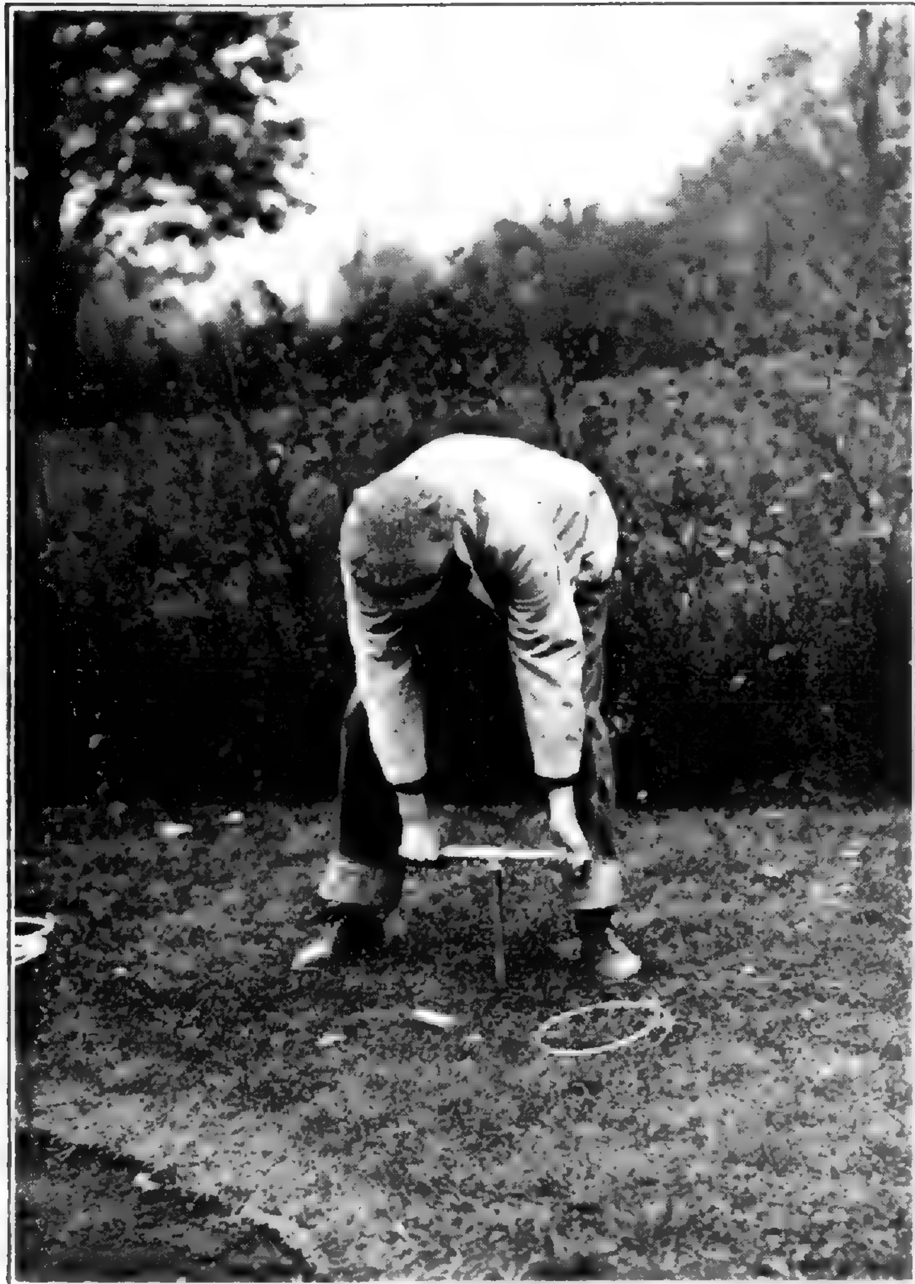
WORK OF VOCATIONAL STUDENTS. Boring holes for dynamite and placing charge.
