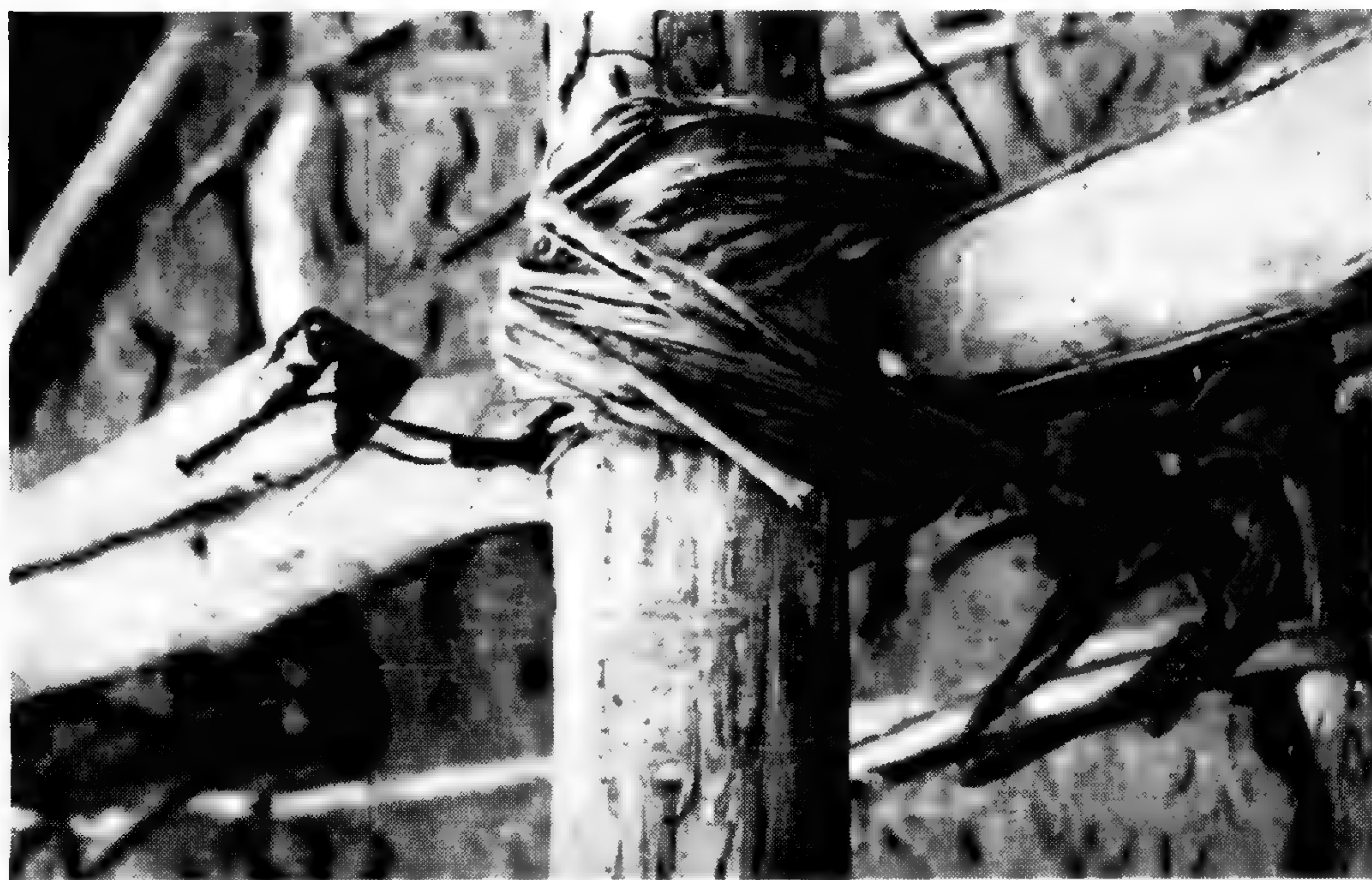
Fig. 1. Cross-beam in a Brazilian hut lashed to an upright by strips of Helicteres bark ( sacarolba ).
