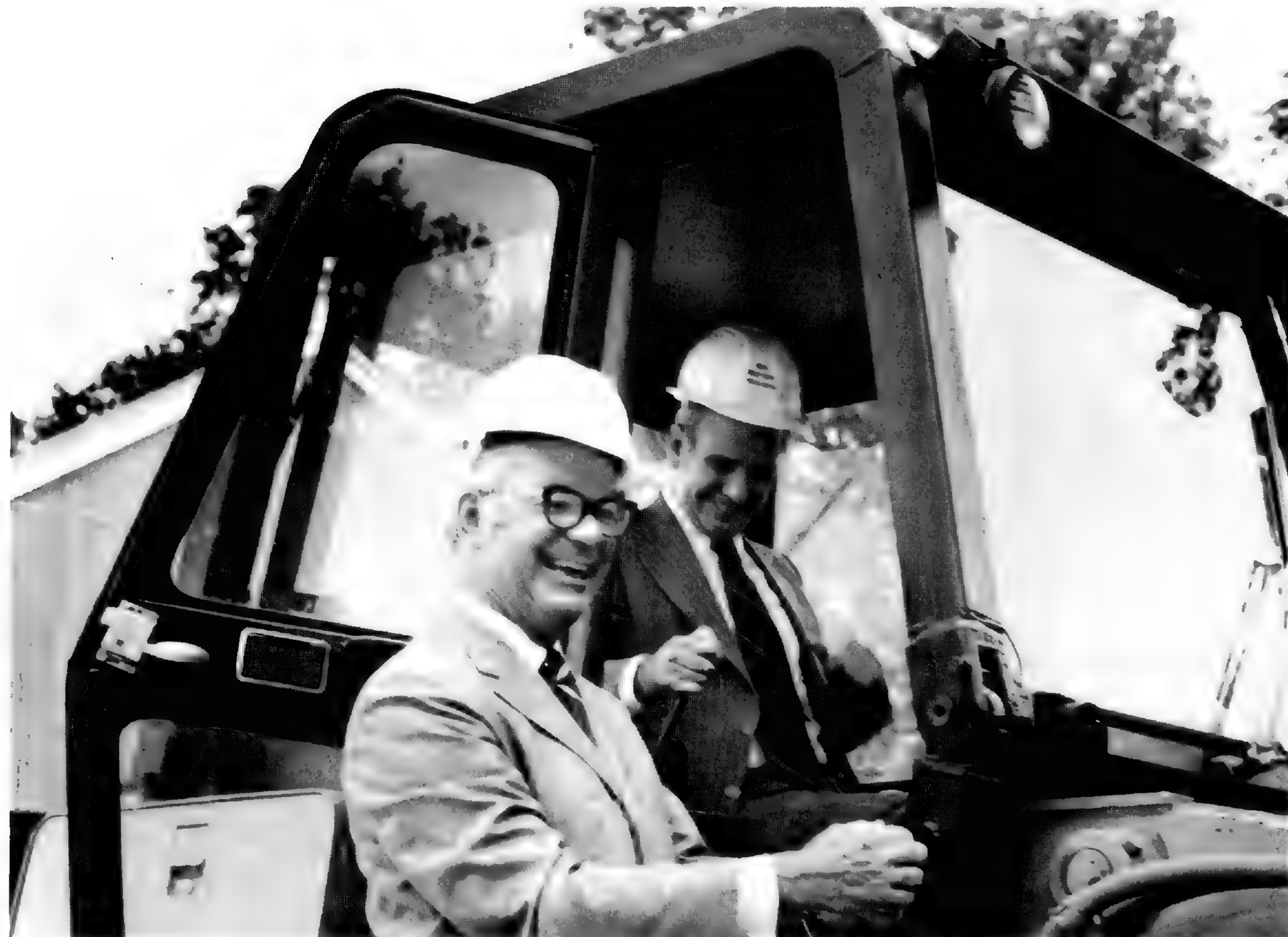
Tom K. Smith, Jr., left, president of the Garden Board of Trustees, and Dr. Peter H. Raven, Garden director, handle heavy equipment to break ground for the new $1 million complex of maintenance buildings.
