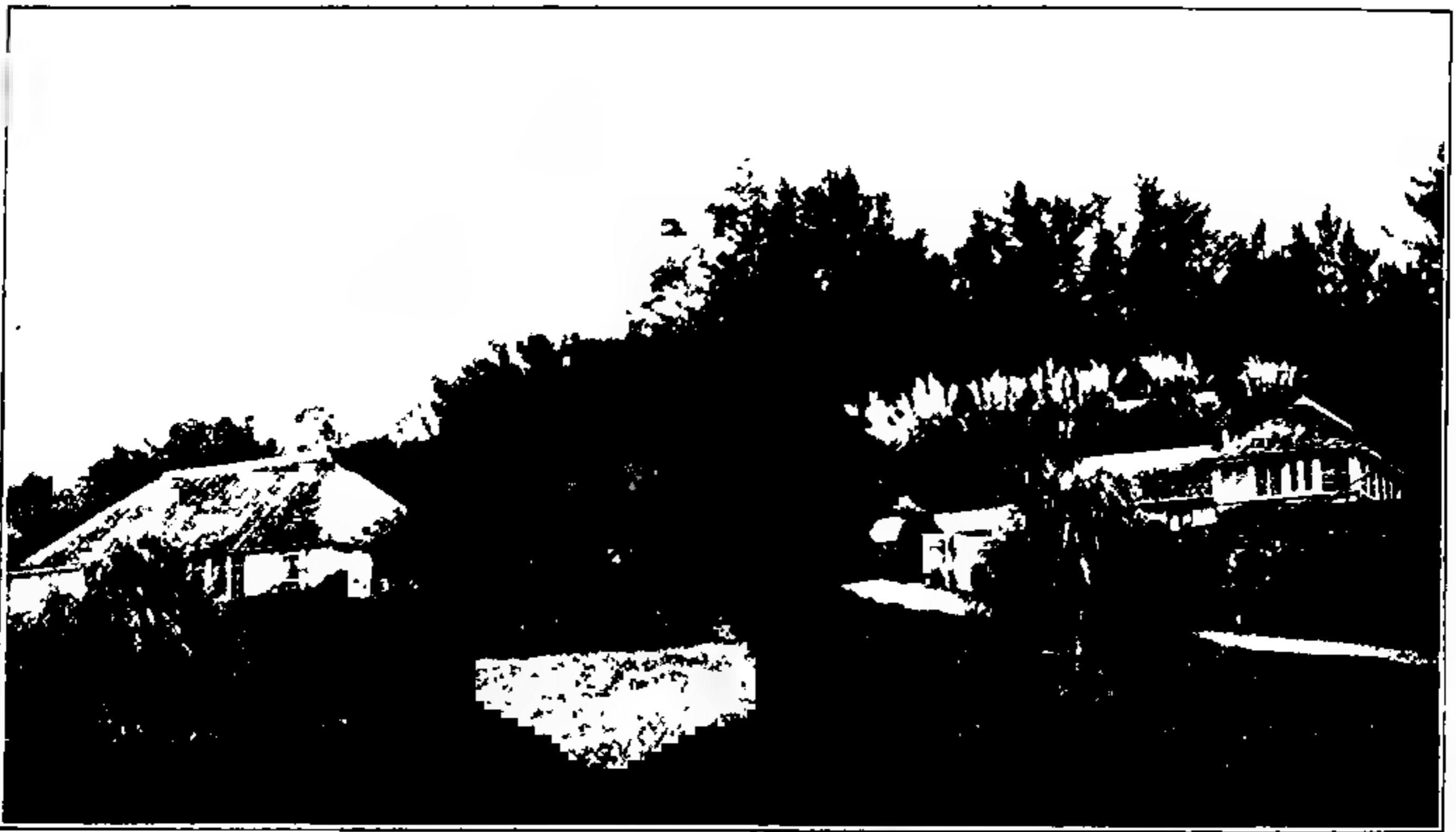
FIG. 7. View of Cinchona, showing the principal buildings. The laboratory is in the background almost concealed by clumps of pampas-grass. Photographed by Dr. Forrest Shreve.
