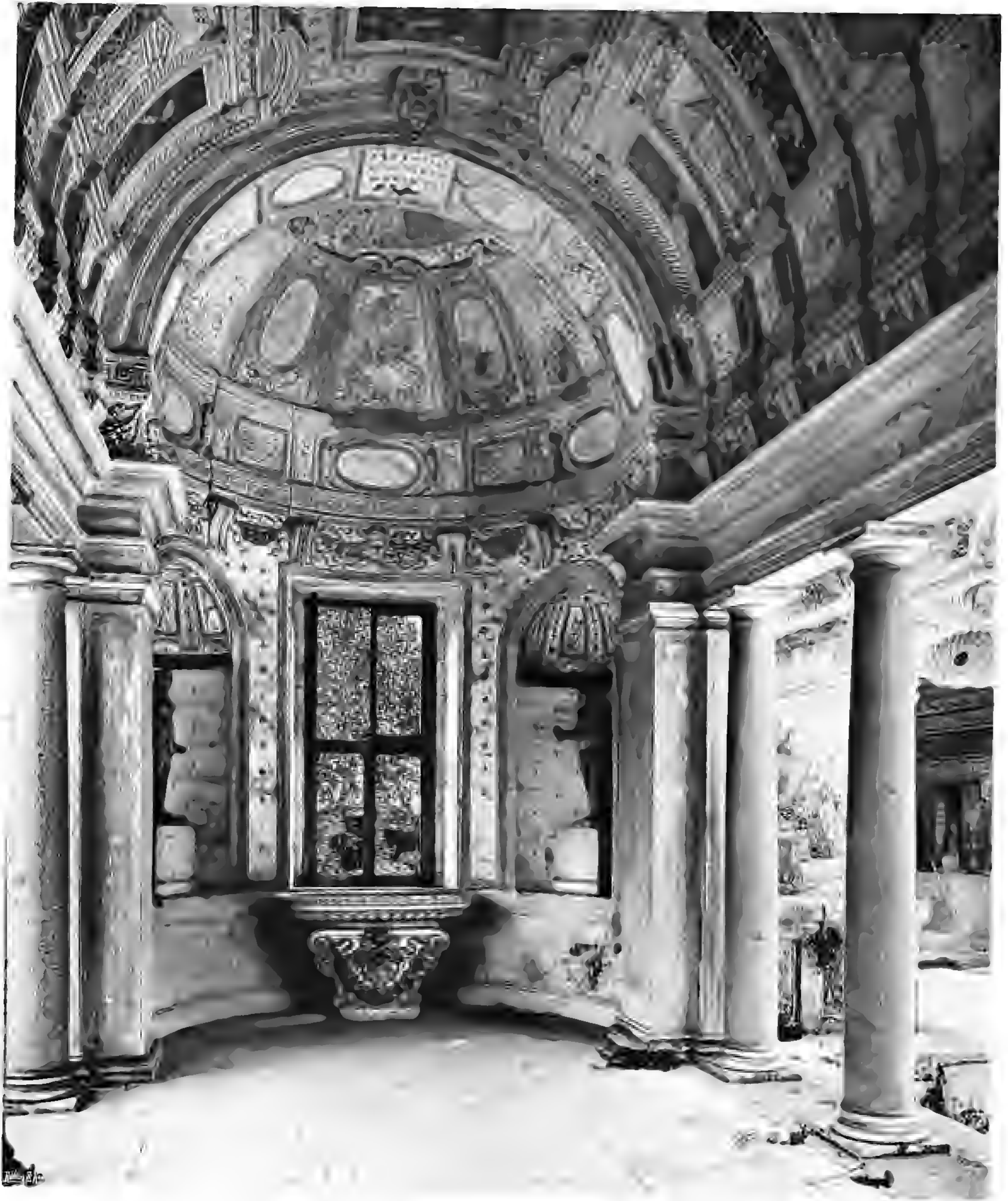
VESTIBUL OF EAST PAVILION—LOOKING SOUTH.
