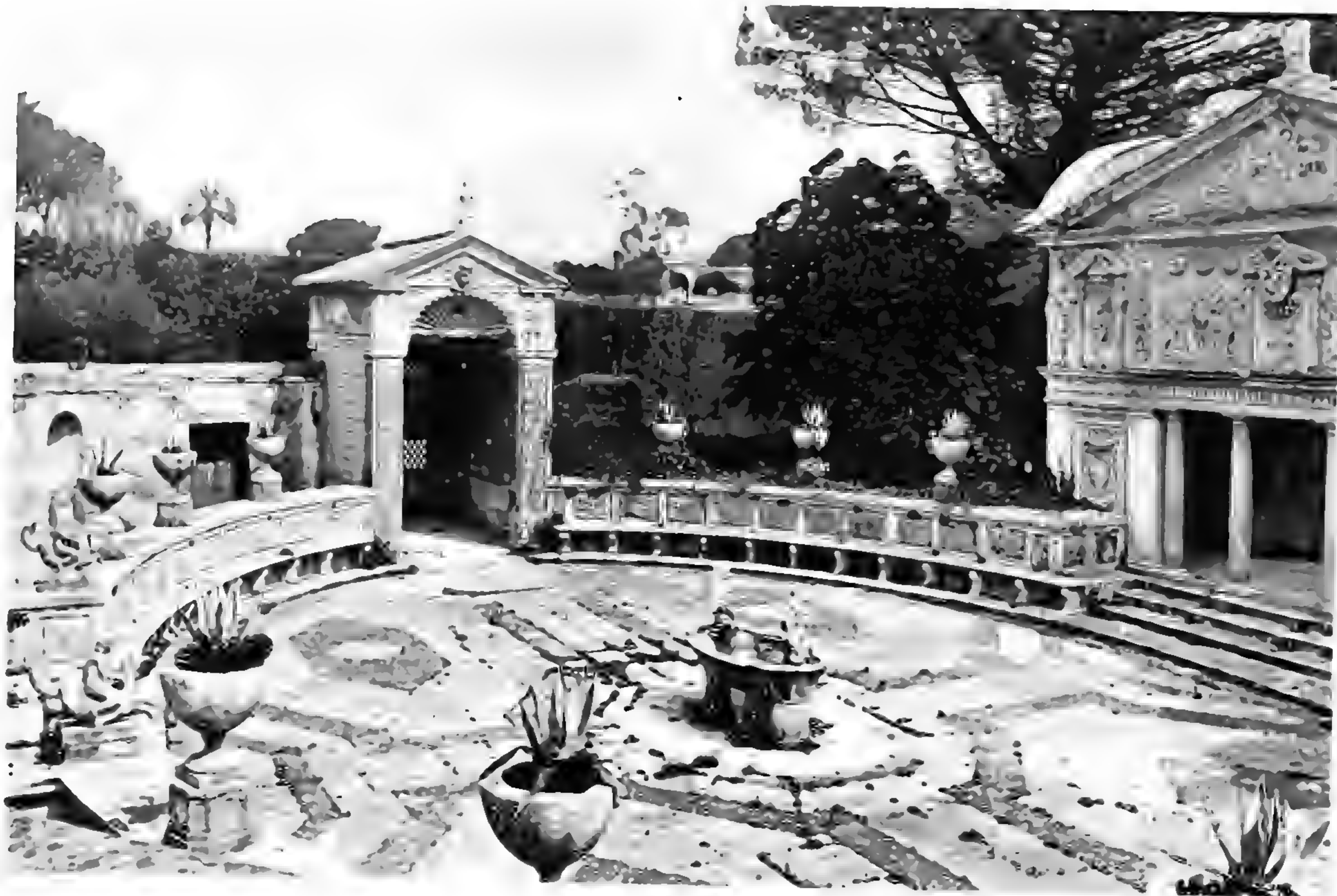
COURT OF VILLINO MEDICI FROM THE SOUTH-WEST.
