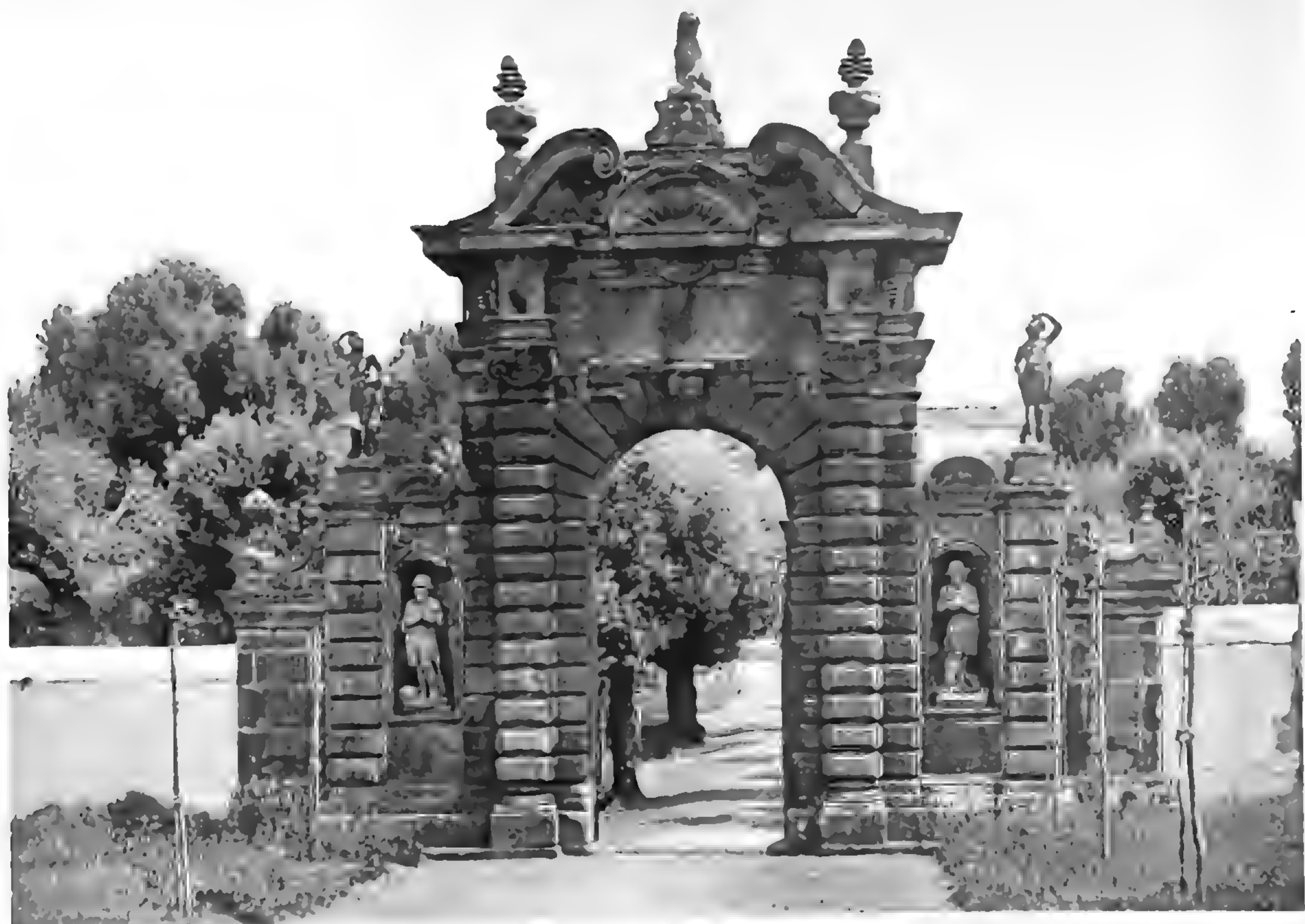
ENTRANCE GATEWAY, SOUTH FRONT.
