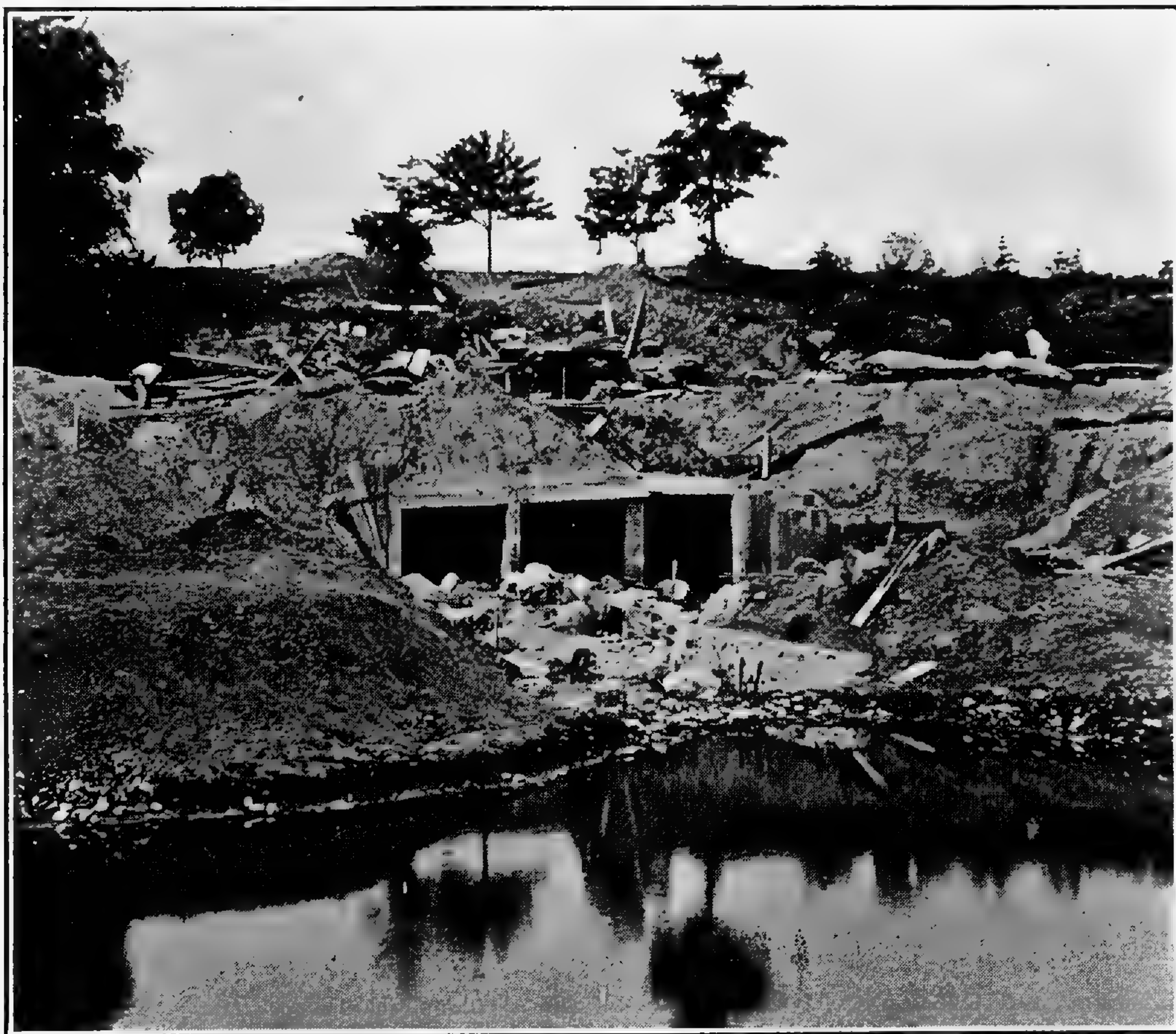
FIG. 5. Japanese garden. Construction of resonating caves for waterfalls. August 18, 1914.
