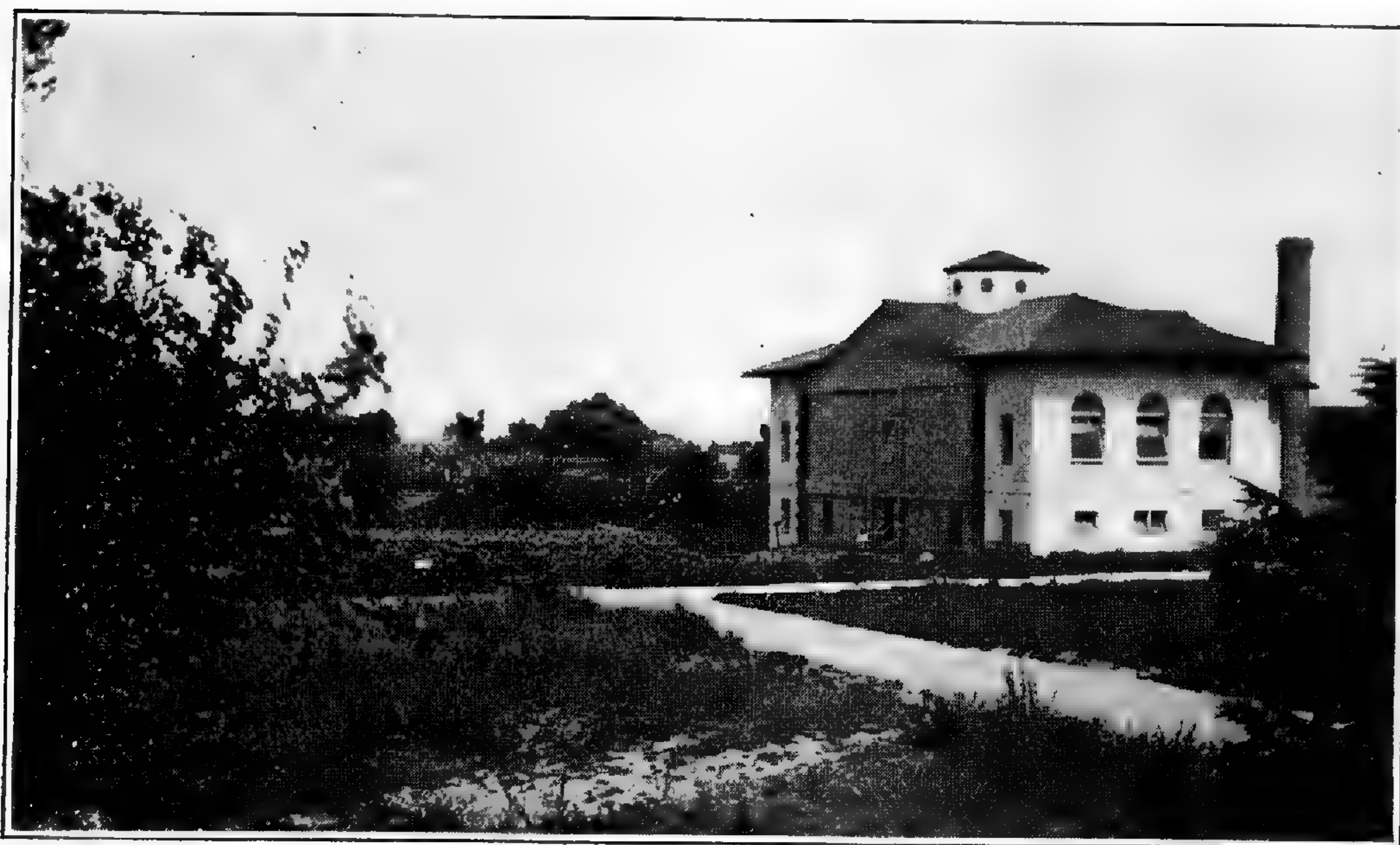
FIG. 2. Laboratory building, summer, 1915. View from the Garden, showing first (south) section, completed September, 1913; at the left, site of the new sections nearing completion in December, 1916. (Cf. Fig. 1.)
