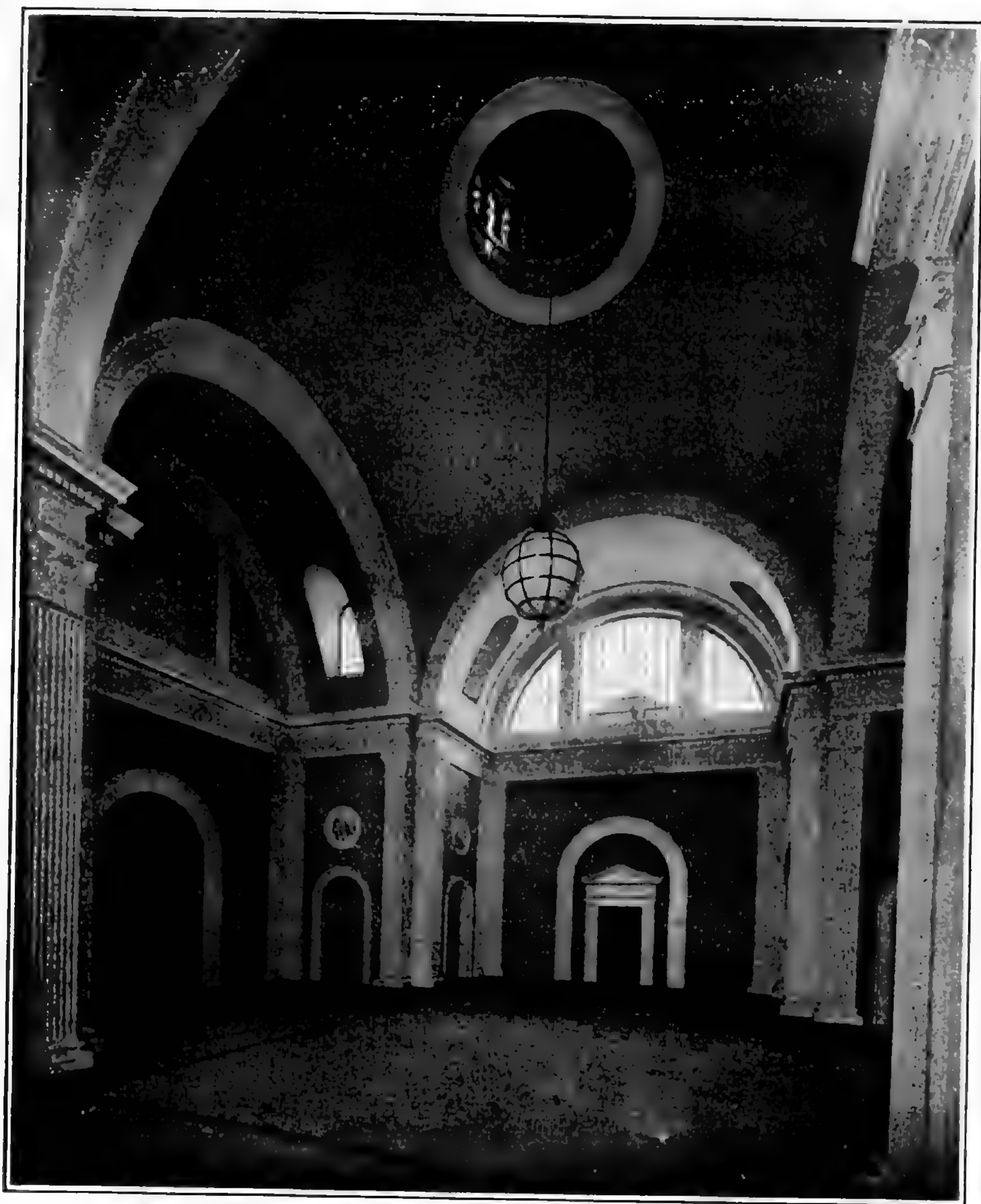
FIG. 9. The central rotunda, main floor, of the laboratory building. View facing east, toward the main entrance to the library. The height from the floor to the opening in the ceiling is 36 feet, 6 inches; to the top of the balustrade, 41 feet.
