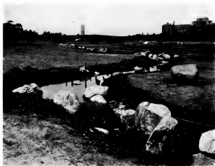
FIG. 8. Glacial boulders placed along the Brook under construction, 1912. (562)
