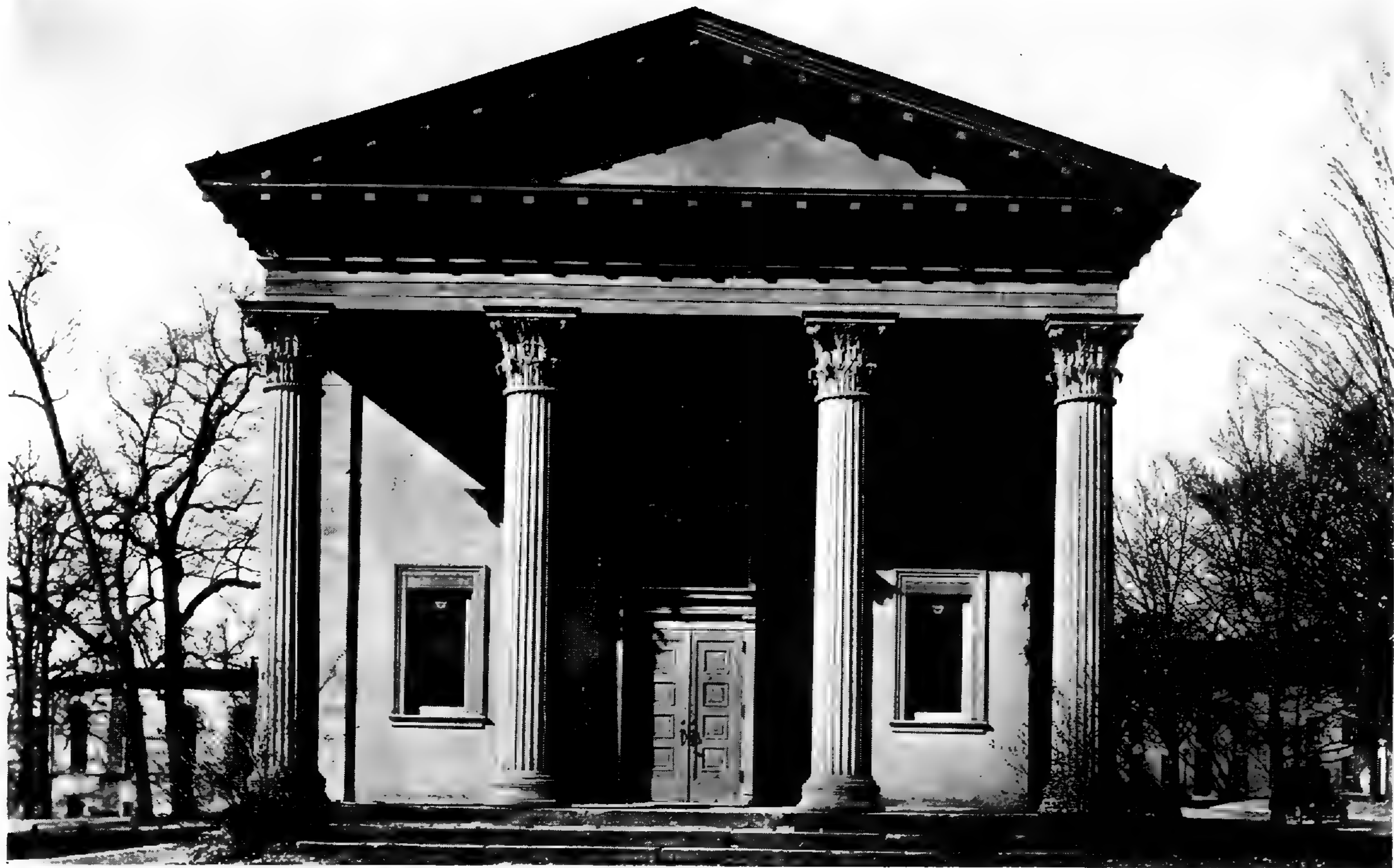
FIG. 15. Corn capitals on the Playmakers' Building, University of North Carolina, Chapel Hill. Designed about 1850 by Alexander J. Davis (cf. Fig. 12). (Courtesy, University of North Carolina.)
