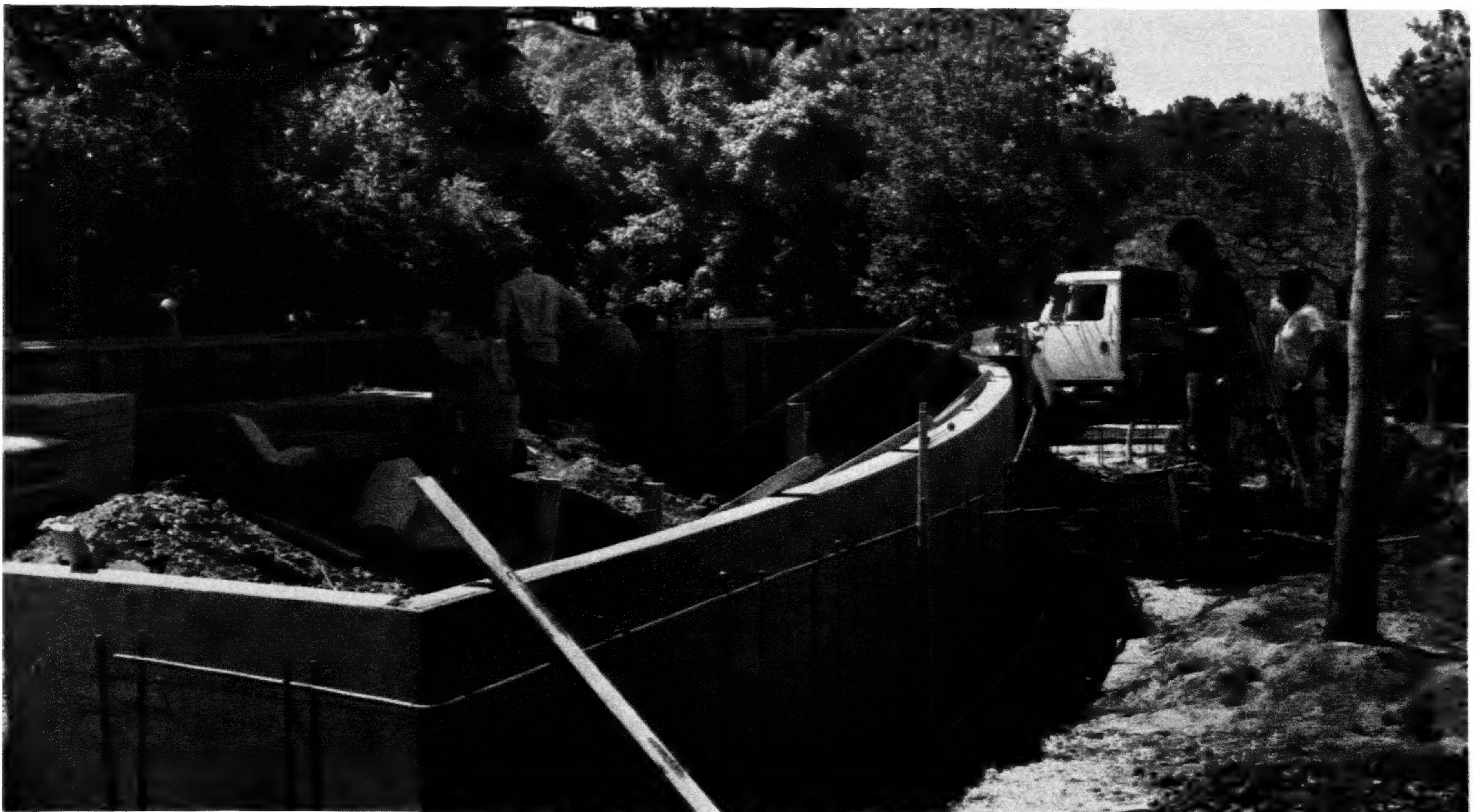
Concrete walls will buttress dining terraces when renovation of the Peacock Cafe is completed in late summer.
