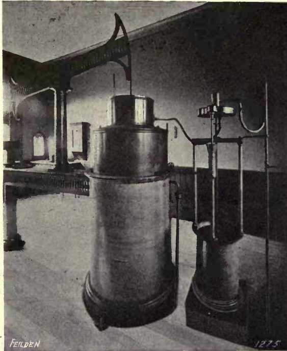
FIG. 88.—BRADDOCK'S PATENT 30-IN. DIAMETER COMPENSATING STATION GOVERNOR, WITH AUTOMATIC SELF-LOADING ARRANGEMENT, AT THE EFFINGHAM-STREET GASWORKS, SHEFFIELD.
