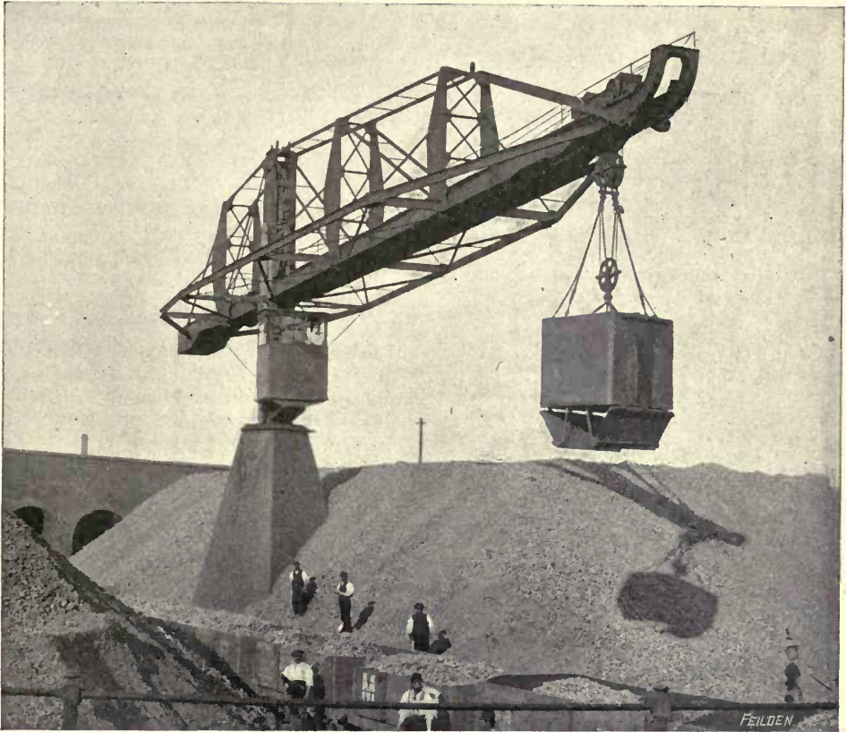
FIG. 33.—HYDRAULIC CRANE FOR STACKING AND LOADING COKE, SALTLEY WORKS, BIRMINGHAM.
