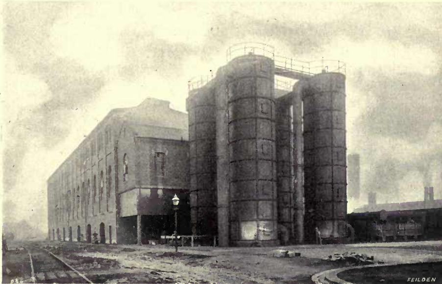
FIG. 50.—WASHERS AND SCRUBBERS AT THE GRIMESTHORPE STATION OF THE SHEFFIELD GAS COMPANY.
