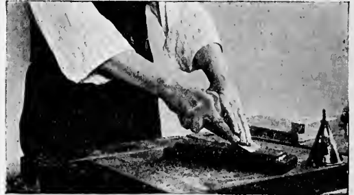
2. Sharpening on Oilstone.
