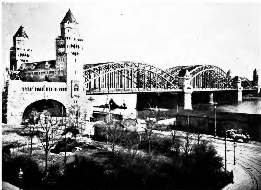
HEAVY TRAFFIC BRIDGE AT COLOGNE
