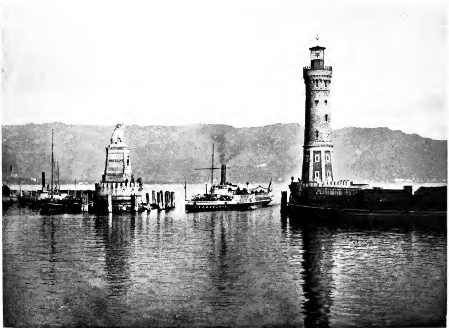
HARBOR GATE, LINDAU Tower and monument form an interesting disymmetric contrast
