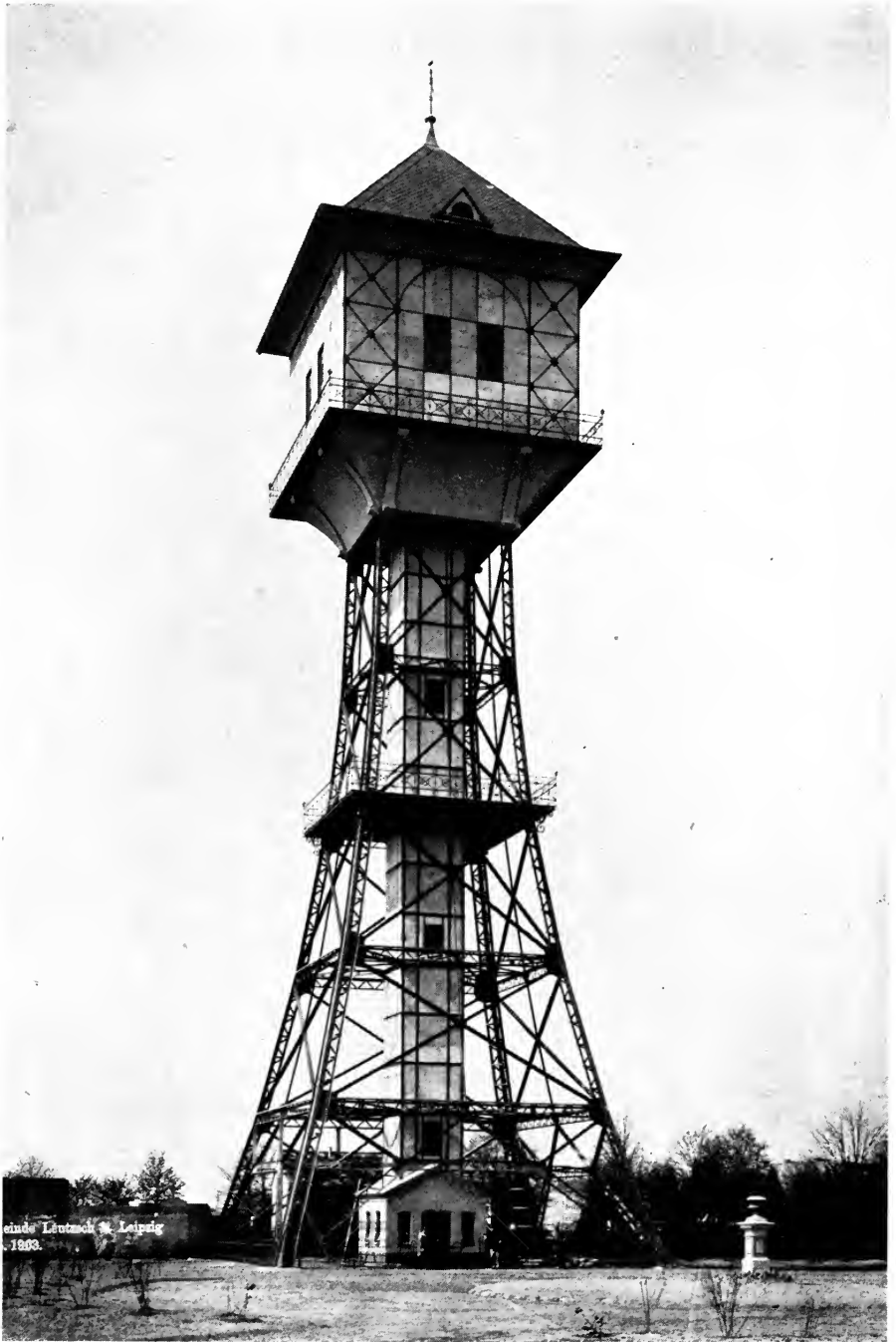
WATERWORKS AT LEUTZSCH, NEAR LEIPZIG 80,000 gallons capacity, 100 feet high
