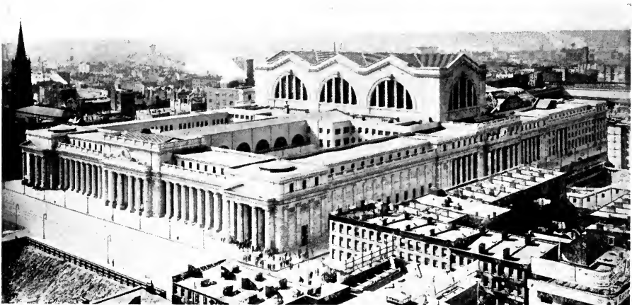
NEW AND TYPICAL AMERICAN RAILWAY STATIONS Union Station, Washington, D. C., Grand Central Station, New York, and the Pennsylvania Station, New York
