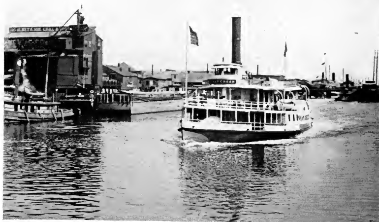
A PART OF THE LOWER HARBOR PROVIDENCE HARBOR
