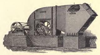
Flg. 160. Hot-Blast Apparatus with Double Duct for Supplying Air at Different Temperatures to Different Parts of a Building.
