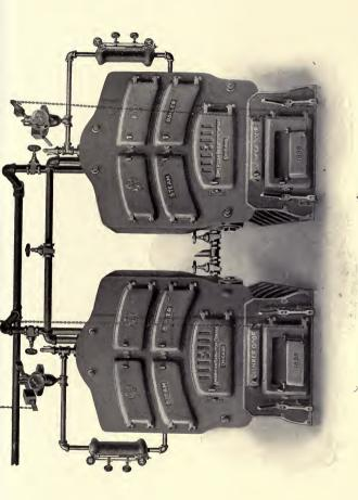
A BATTERY OF IDEAL STEAM BUILERS SHOWING METHOD OF YOKING THE MAIN SUPPLY AND RETURN FIPE. American Radiator Company.
