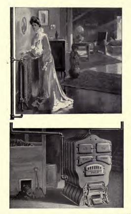
TYPICAL HEATING INSTALLATION SHOWING SECTIONAL BOILER AND RADIATOR. American Radiator Company.
