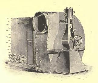
Fig. 144. Combined Heater and Centrifugal Fan with Direct-Connected Engine.
