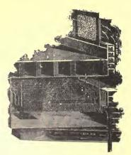
Fig. 51. Steam Heater Connected to Wall Register.—Indirect System.
