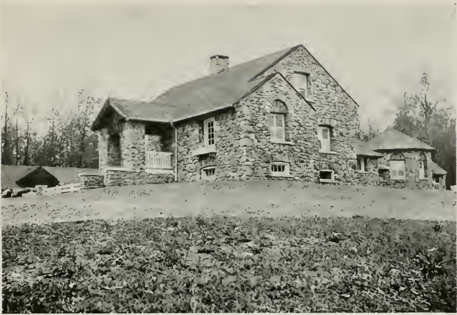
A GOOD GROUPING BUT SADLY IN-NEED OF PLANTING. FARM BUILDINGS FOR CHARLES E. RUSHMORE, ESQ., WOODBURY FALLS, N. Y.
