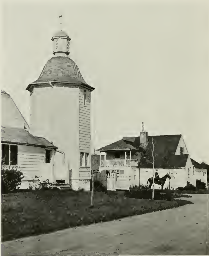
THE TOWER. FARM BUILDINGS FOR J. E. DAVIS, ESQ., BROOKVILLE, L. I.
