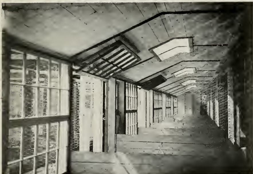
THE INTERIOR OF A CHICKEN HOUSE. THE LARGE WINDOWS FOLD IN THE CENTER AND ARE HOOKED UP AGAINST THE CEILING
