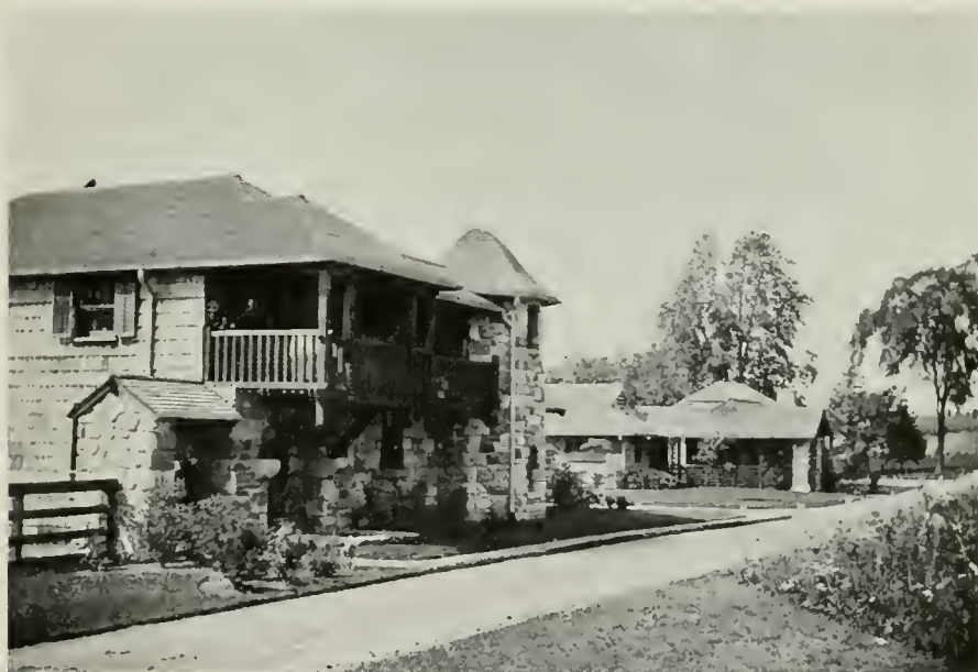
FARM BUILDINGS FOR H. F. FISHER, ESQ., GREENWICH, CONN.
