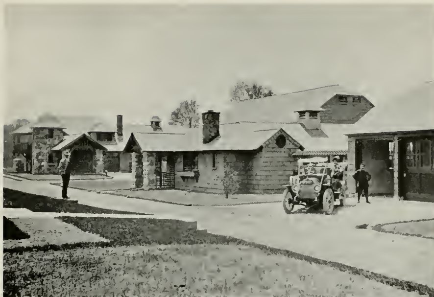
INTERESTING GROUPING AND GOOD ROOF LINES. RIVED SHINGLES FOR WALLS, WITH PORTION OF BUILDINGS OF FIELD STONE. THIS PHOTOGRAPH WAS TAKEN BEFORE THE PLANTING WAS STARTED
