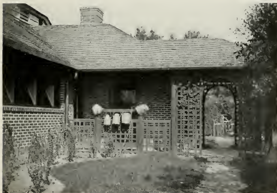
THE DAIRY. FARM BUILDINGS FOR S. T. PETERS, ESQ., ISLIP, L. I.
