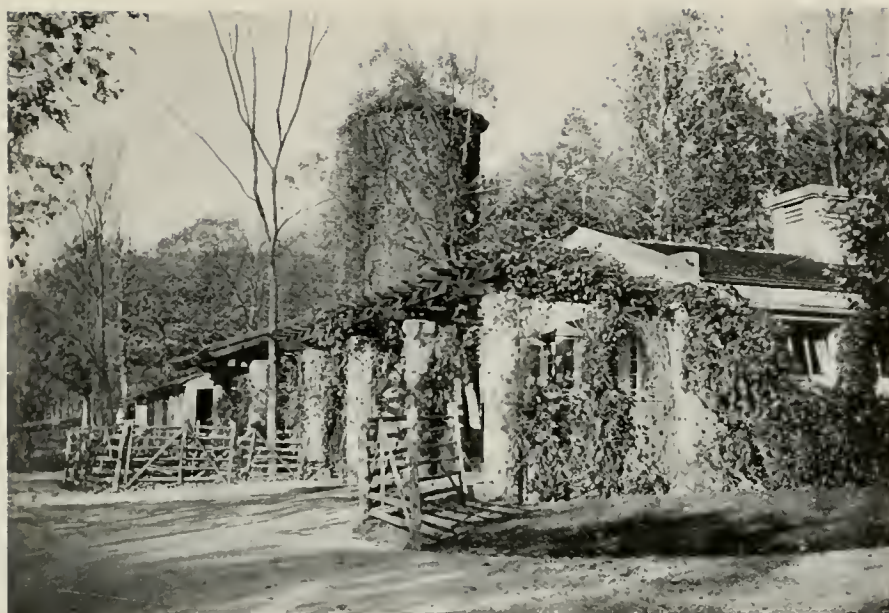
THE LARGE POSTS WITH RAFTERS ABOVE SUPPORT THE MANURE TROLLEY
