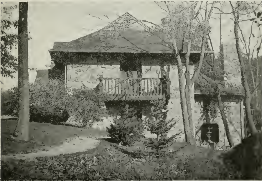
ROUGH FIELD STONE AND HEWN TIMBERS. COACH STABLE AND COACHMAN'S COTTAGE FOR FRANCIS LYNDE STETSON, ESQ., STERLINGTON, N. Y.
