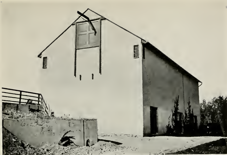
SHOWING THE METHOD OF SLIDING THE HAY DOOR WHEN THIS IS LOCATED NEAR THE RIDGE. THE TWO LOUVERS AT THE EAVES ARE AT THE TOP OF THE VENTILATING DUCTS FROM THE ROOT CELLAR BELOW
