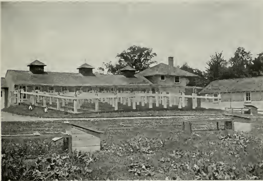
YARDS AND BROODER HOUSE; STORAGE SHED AT RIGHT. CHICKEN HOUSES FOR FRANCIS LYNDE STETSON, ESQ., STERLINGTON, N. Y.
