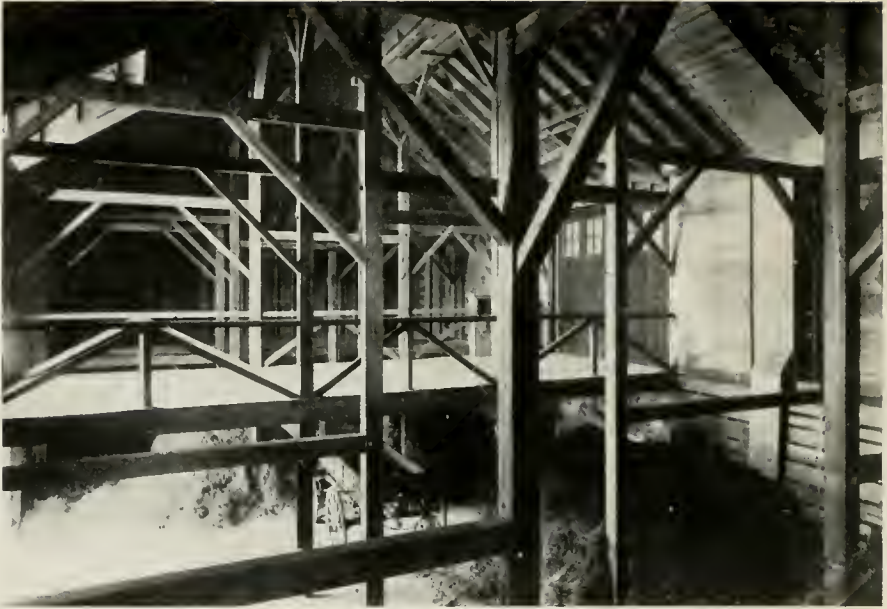
THE FARMER'S METHOD OF FRAMING THE HAY BARN
