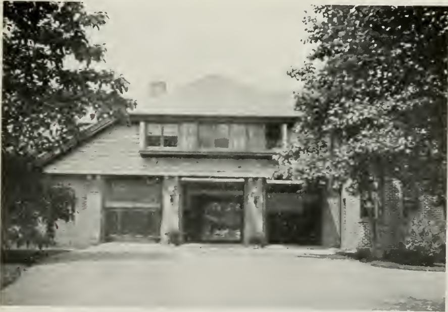
SHOWING ENTRANCE DOORS TO GARAGE FOR S. T. PETERS, ESQ., ISLIP, L. I.
