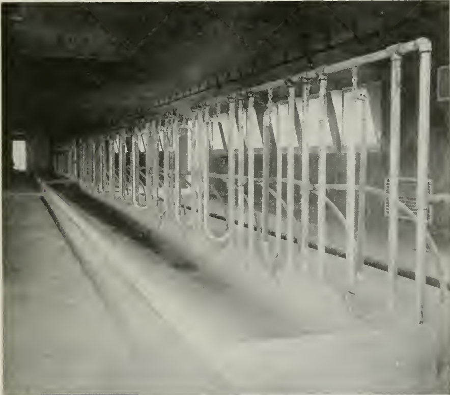
COW BARN INTERIOR, SHOWING STEEL STANCHIONS AND ALSO AN EXCELLENT TYPE OF THE FEEDING-TROUGH—LOW AND BROAD
