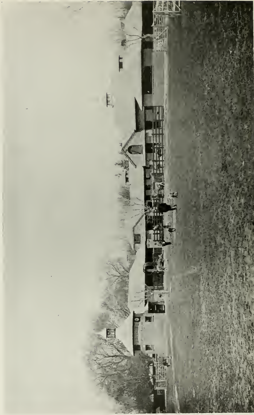
AN INTERESTING GROUPING IN WHICH THE ROOF LINES WERE SOFTENED BY ROUNDING THE HIPS AND RIDGES, FARM BUILDINGS FOR S. T. PETERS, ESQ., ISLIP, L. I.
