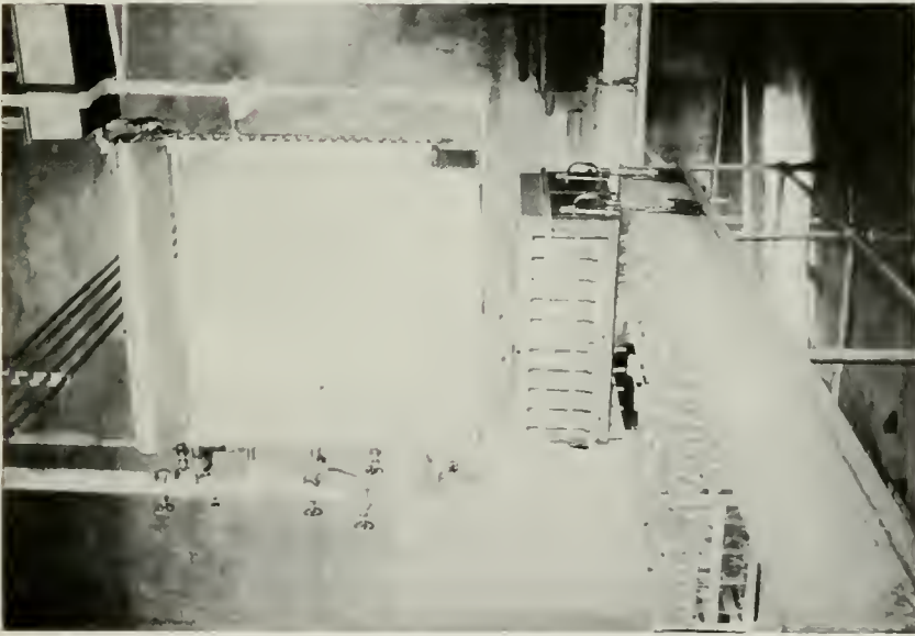
LARGE MILK COOLER FOR COMMERCIAL PLANT, BOTTLING-TABLE WITH HIGH SIDES FOR PACKING BOTTLES IN ICE
