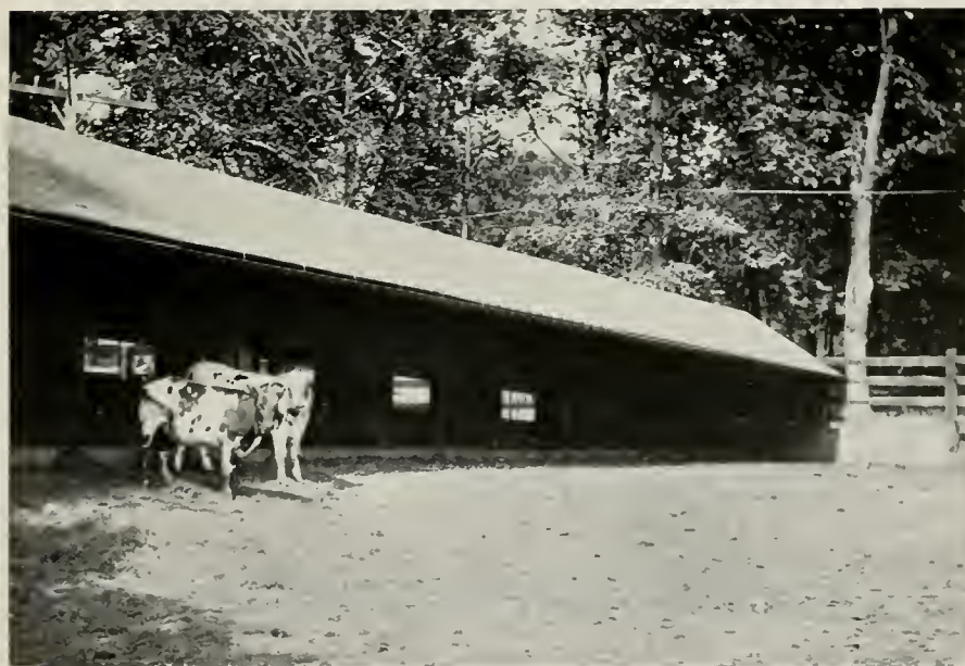
SHELTER AT NORTH END OF COW YARD. FARM BUILDINGS FOR FRANCIS LYNDE STETSON, ESQ., STERLINGTON, N. Y.
