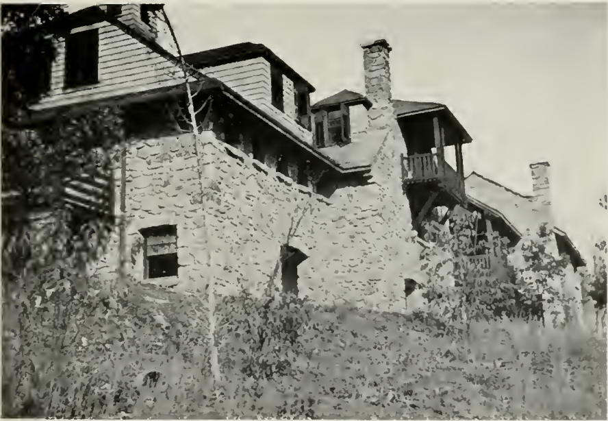
THE BROKEN ROOF LINES AT THE BACK. STABLE AND GARAGE FOR C. R. AGNEW, ESQ., ARMONK, N. Y.
