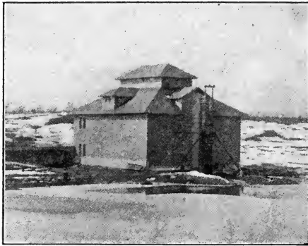
Fig. 79.—LOCAL COLD STORAGE
