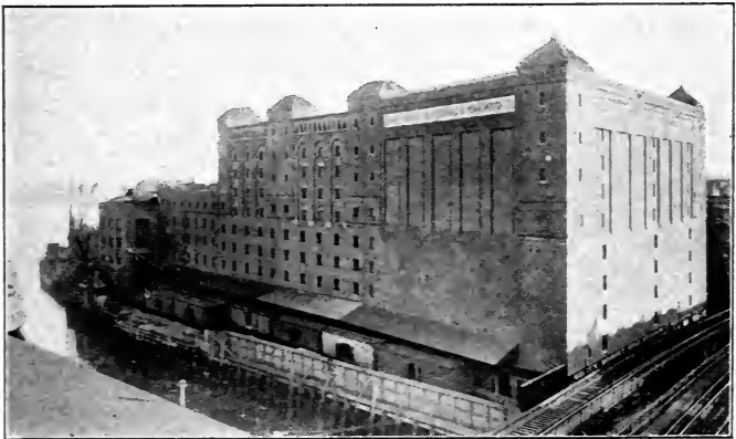
Fig. 80.—A LARGE PUBLIC COLD STORAGE
