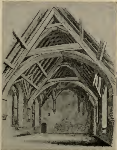
INTERIOR OF THE HALL OF STOKE CASTLE.
