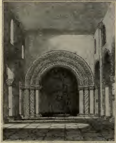
NORMAN DOORWAY, St. Peters, Northampton.—From Old England . (Note the massive round arch and the simple but effective ornament.)
