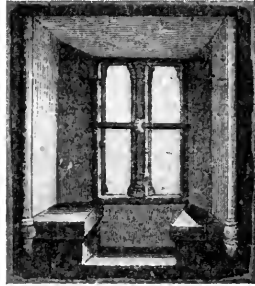
INTERIOR VIEW OF THE UPPER WINDOW SHOWN IN MELICHOPE MANOR HOUSE. This view shows the depth of the wall, — into which, indeed, the stairway is cut.
