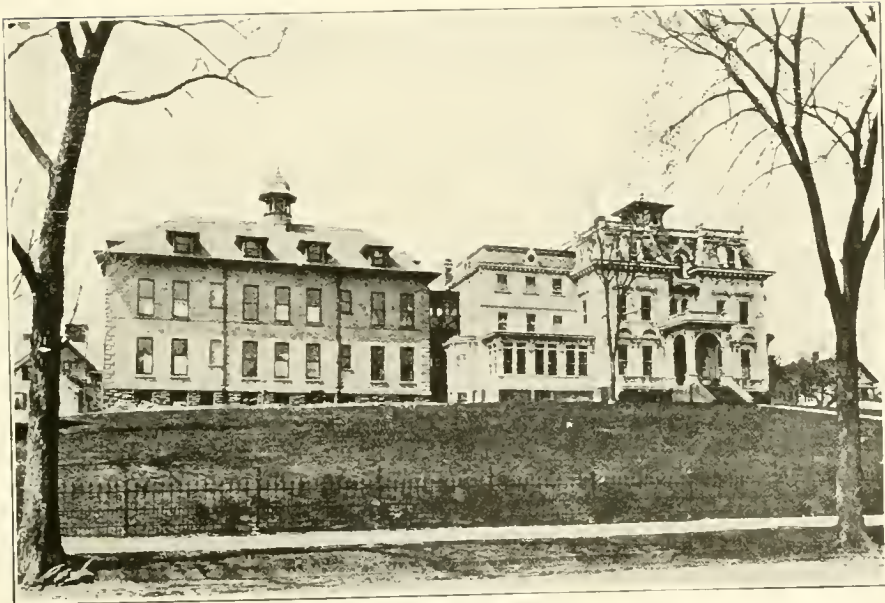
MERIDEN HOSPITAL, MERIDEN
