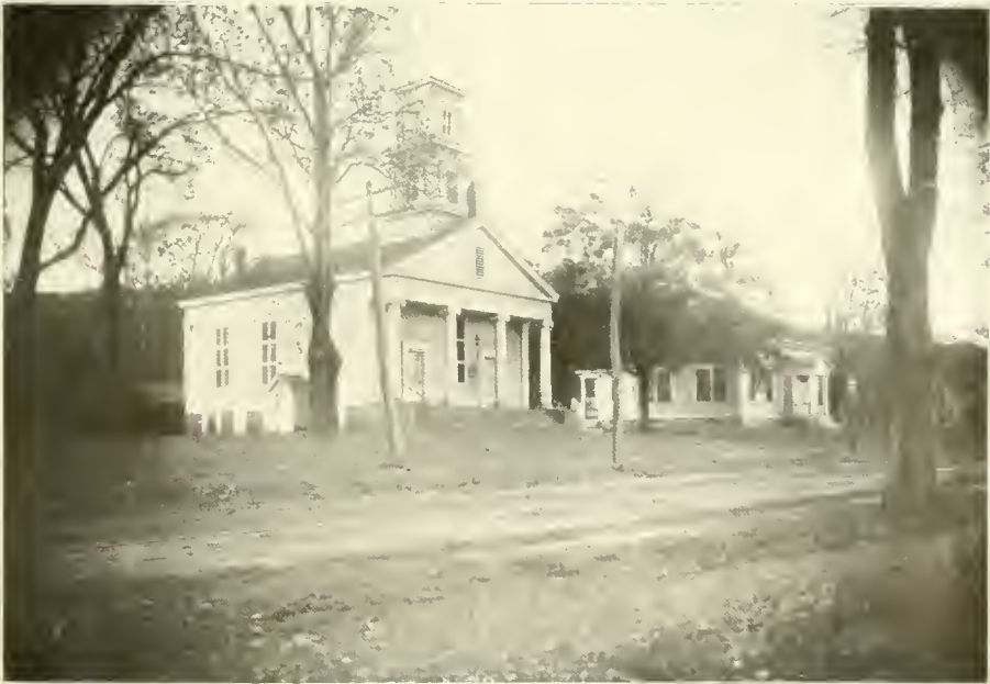
CONGREGATIONAL CHURCH AND PARISH HOUSE, MOUNT CARMEL
