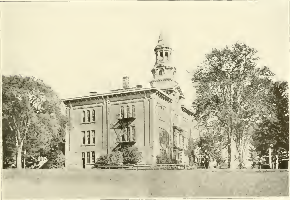
HIGH SCHOOL BUILDING, WALLINGFORD
