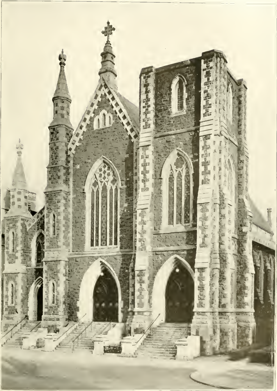
ST. MARY'S ROMAN CATHOLIC CHURCH, NEW HAVEN
