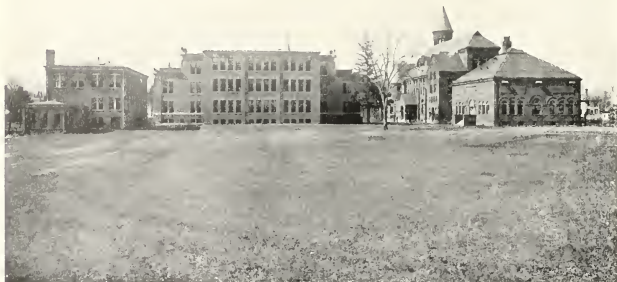
FREE ACADEMY—ABOVE, AT LEFT, SLATER HALL, LIBRARY AND MUSEUM, WITH ART DEPARTMENT IN REAR, IN CENTER, MAIN ACADEMY BUILDING. BELOW, REAR VIEW; AT LEFT, MANUAL TRAINING BUILDING; CENTER, MAIN ACADEMY BUILDING; AT RIGHT, SLATER HALL SHOWING ART BUILDING.
