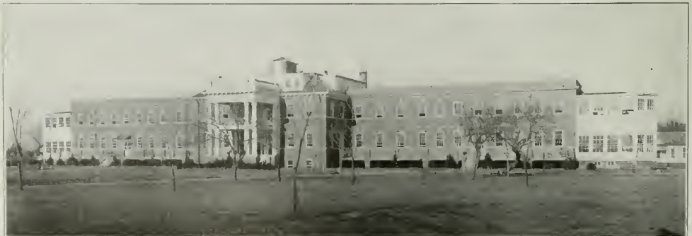
The Municipal Tuberculosis Hospital, at Trenton, N. J., is one of the hospitals opened in 1920. Wm. A. Klemann, architect, Trenton, N. J.
