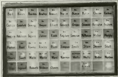
Fig. 2. This device, located on the wall by the telephone switchboard, indicates by the light whether or not the physician is in the hospital.
