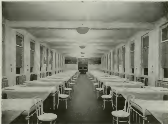
Fig. 5. The soft, comfortable lighting produced by the indirect system is shown in this view of a ward of oblong shape using a single row of outlets. The cords for the signal system will be noted between the beds at each side of the room.
