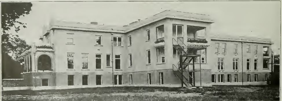
The Good Samaritan Hospital of Sandusky, Ohio, is built in the shape of a cross, thus dividing the building into four distinct departments, all of which are accessible from the center of the building. The northern projection on the first floor is used for offices, reception rooms, staff room, etc., and on the second floor for the operating department. In the east and west projections are patients' rooms, all on the south side, the side toward the center being used for all the utilities, including the kitchens, elevators, etc. There is an isolation department on the first floor, connecting with a special exit on the south side. Stevens and Lee, architects, Boston.
