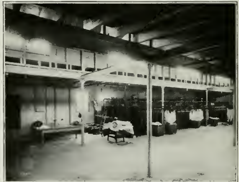
LARGE CONVEYOR DRYROOMS.
