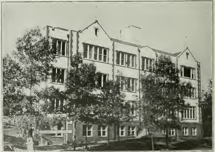
The Salvation Army Hospital and Home at Greenville, S. C., is an institution that has been built for the treating of women and children in the district of the Southeast, comprising the states of North Carolina, South Carolina, Florida and Georgia. The new hospital is modern in every particular, the construction of the main building being of reinforced concrete and hollow tile, fire proof throughout, and the latest types of operating, refrigerating, sterilizing, kitchen, and laundry equipment being provided. Beacham and LeGrand, Greenville, S. C., architects.
