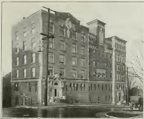
The Virginia Mason Hospital, Seattle Washington, just completed by a group of Seattle physicians, is built on a hill above the city so that it has a view over the city and Puget Sound off to the mountains. The main floor entrance opens into a large waiting room attractively furnished in grey wicker and blue tapestry. A main office connects with the waiting room and a wide corridor leads to the offices of the various doctors. The hospital entrance and waiting room are on the floor below, made possible by the grade on which the building is situated. The second, third, and fourth floors are given over to the patients' rooms, having sixty beds, while on the sixth floor is the operating suite, sterilizing rooms, rest rooms, and nurses' quarters. Bebb and Gould, architects, Seattle, Wash.
