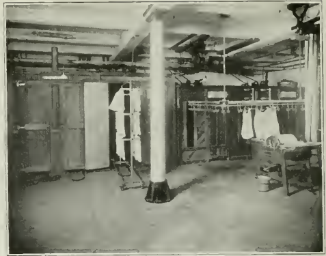
VIEW OF DRYROOMS.
