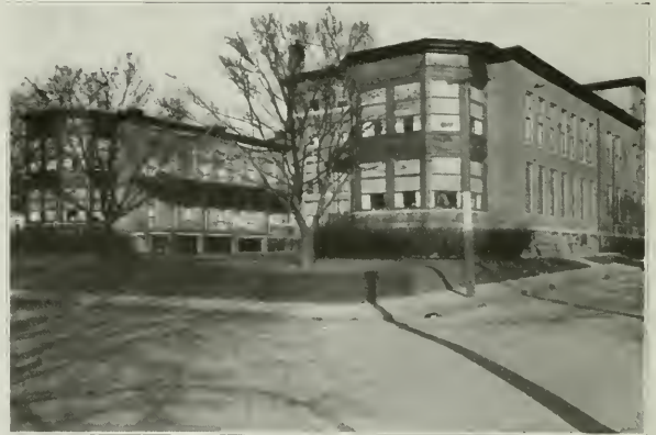
Front view of the Union Hospital, Fall River, Mass. Stevens Clinic stands just back of these buildings.
