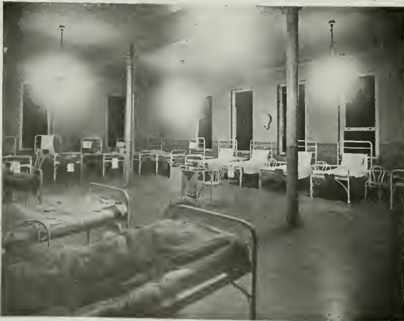
Fig. 6. Enclosing glassware which diffuses the light and which can be readily cleaned is used in this square-shaped ward for general illumination. Such lighting is simple of installation, inexpensive and a remarkable improvement over much of the equipment now in use.
