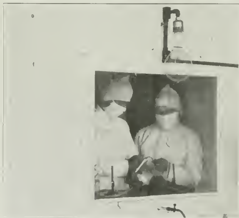
Bacteriological workroom, showing exterior, with operators inside seen through the plate glass, sealed window. The room is plastered throughout on the inside, is provided with a high pressure sprinkler, which washes down every part of it, and is supplied with air, filtered through cotton.
