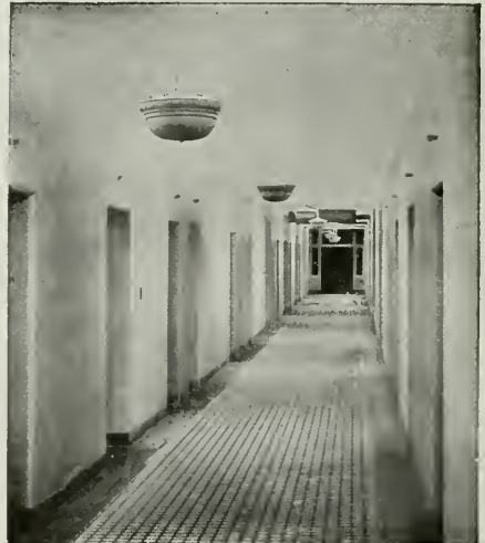
Fig. 3. A corridor illuminated by the totally indirect system. Fixtures are placed approximately twenty-one feet apart and one-half watt per square foot of floor area is provided. The glass cover above the reflector should be noted, making it a very simple matter to clean and maintain fixtures in a sanitary condition.
