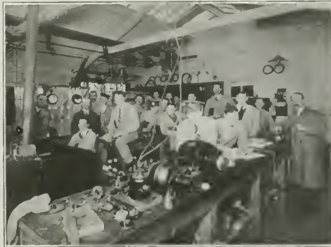
Electrical workshop at Roehampton.
