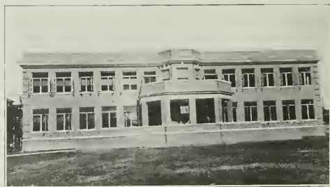
Rear view of the Hofheimer Children's Building of the Memorial Jewish Hospital for Consumptives.
