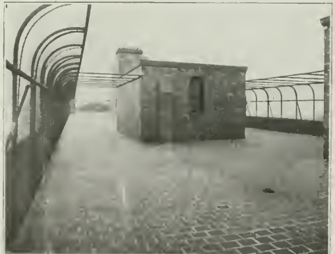
This photograph from the Mercy Hospital, Pittsburgh, Pa., shows a development for roof garden purposes, with the recreational facilities as the main object. The elevator, dumb waiter and lavatories are probably in the small covered space. Additional space could easily have been added as a place where patients could be placed for treatment and examination.
