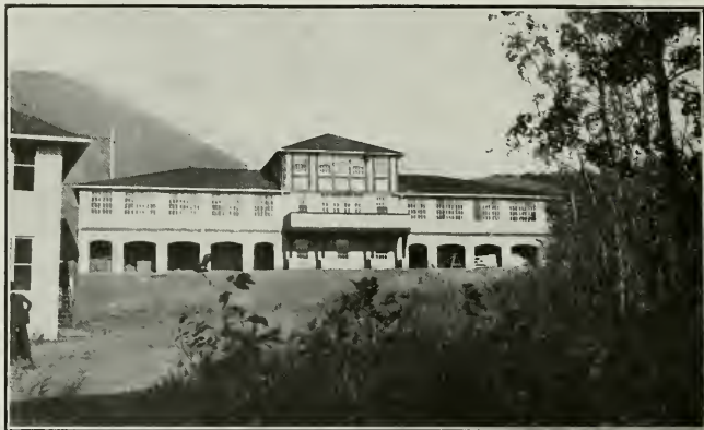
Front View of Children's Pavilion, Saskatchewan Sanatorium.
