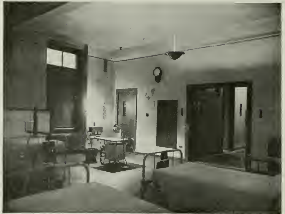
Fig. 7. A semi-private ward lighted by a single porcelain enameled totally indirect unit. The nurse's desk with a local light located near the main control panel will be noted. Baseboard receptacles and emergency lights are properly placed.
