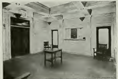
Fig. 1. Night view of a typical well designed hospital lobby illuminated by the indirect method supplemented by wall brackets and local lighting near the elevator. A harmonious and pleasing room is thus provided.
