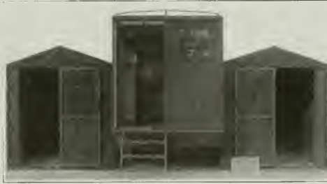
Looking at the mobile dental clinic from the rear. This picture shows the clinic ready for business, with the collapsible wall tents lowered and set up on each side of the truck.
