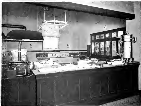
Counter and kitchen of a cafeteria suitable for a small hospital.
