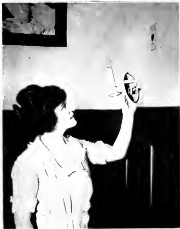
A wall bracket ready to put in place. Note the inconspicuous receptacle above.
