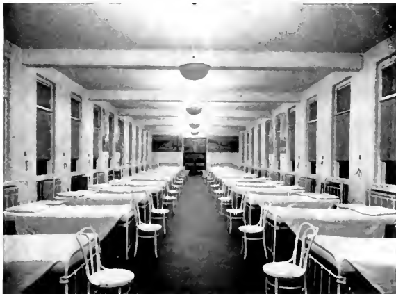
Fig. 5. The soft, comfortable lighting produced by the indirect system is shown in this view of a ward of oblong shape using a single row of outlets. The cords for the signal system will be noted between the beds at each side of the room.
