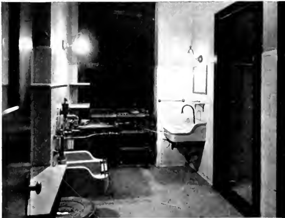
Fig. 8. Night view of a utility room showing the local lighting from bracket units over the sink and sterilizing apparatus. Sufficient light is transmitted through the opalescent reflectors to provide general illumination.
