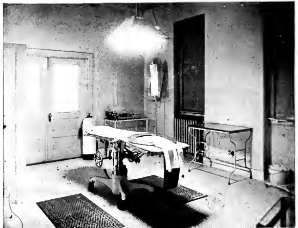
Fig. 11. A diffusing type of operating table fixture equipped with six 100-watt Mazda C lamps in mirrored reflectors. A diffusing glass plate covers the lower side of the unit, which is so constructed as to provide for dissipating the generated heat.
