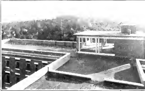
The roof of the Waterbury Hospital, Waterbury, Conn., quite fully illustrates the possibilities of hospital roof service. Here is a large area entirely unused except for slight recreational purposes. The elevator and lavatories are to be found in the enclosed space, and there is a covered space for protection from storms. The larger roof could just as well be used for the enjoyment of the patients, and as a productive part of the hospital.
