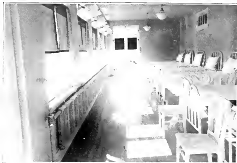
The radiation, ventilation by transoms, indirect lighting, and abundance of sunlight are interesting points in this girls' dormitory.
