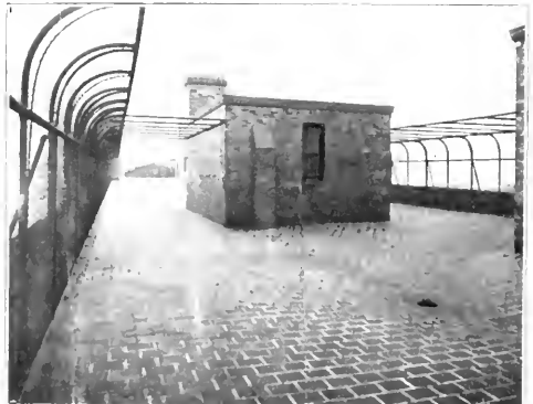
This photograph from the Mercy Hospital, Pittsburgh, Pa., shows a development for roof garden purposes, with the recreational facilities as the main object. The elevator, dumb waiter and lavatories are probably in the small covered space. Additional space could easily have been added as a place where patients could be placed for treatment and examination.
