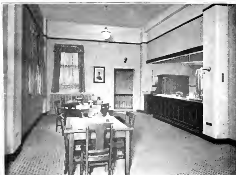
The cafeteria dining room adjacent to the service counter shown above.
