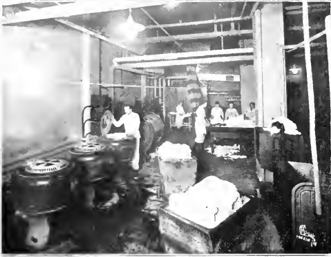
Fig. 4.—Row of Under-driven Extractors.
