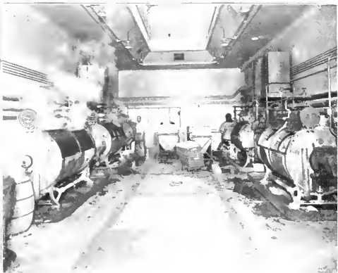
Fig. 5.—Section of a well lighted laundry with ample working space.
