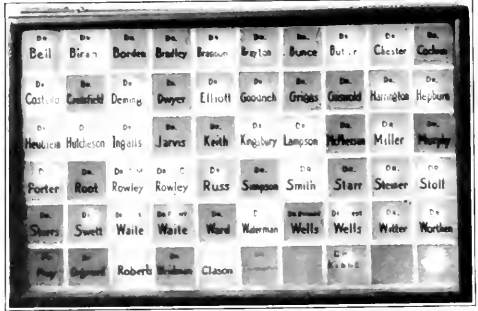
Fig. 2. This device, located on the wall by the telephone switchboard, indicates by the light whether or not the physician is in the hospital.
