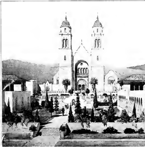
The Chapel, Southern Baptist Sanatorium.
