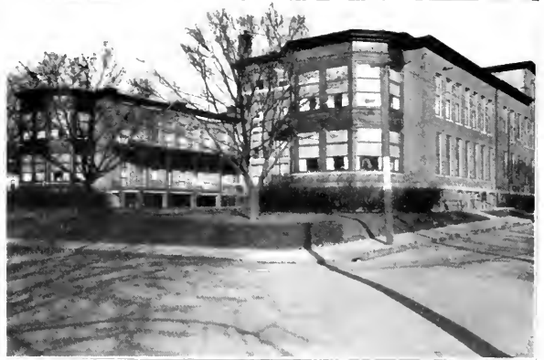
Front view of the Union Hospital, Fall River, Mass. Stevens Clinic stands just back of these buildings.
