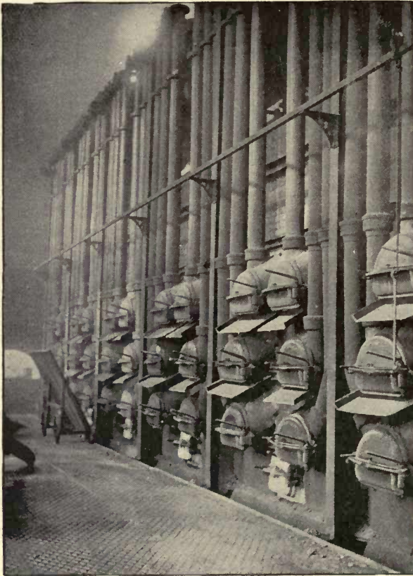
FIG. 17.—VIEW SHOWING COKE SCREEN AND DRAWING STAGE.
