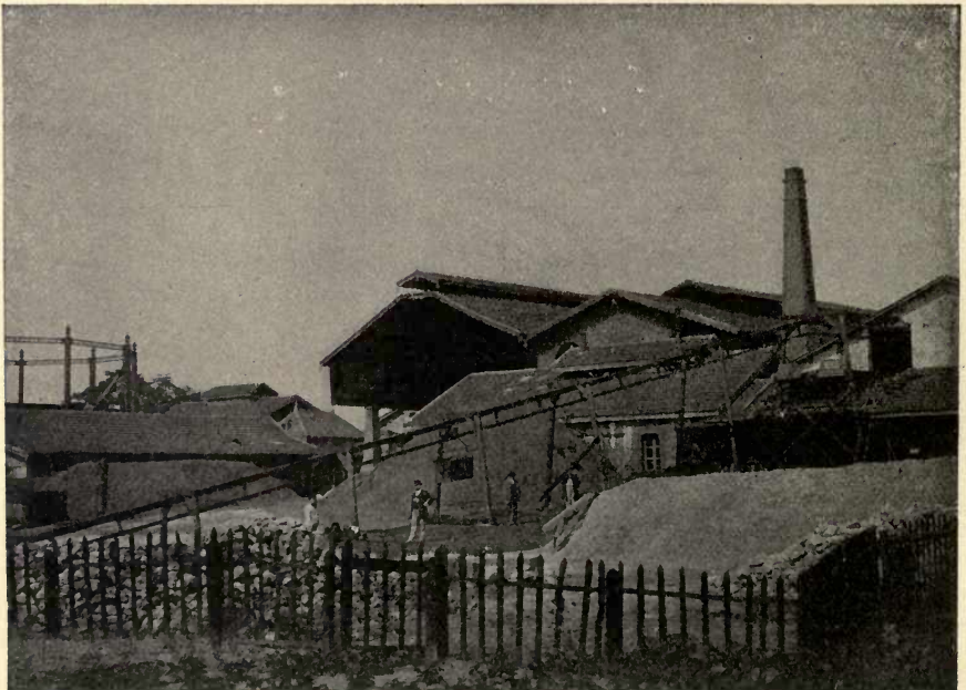
FIG. 1.—VIEW OF THE METZ GASWORKS, SHOWING AERIAL ROPEWAY USED FOR CARRYING COAL TO THE STORES.
