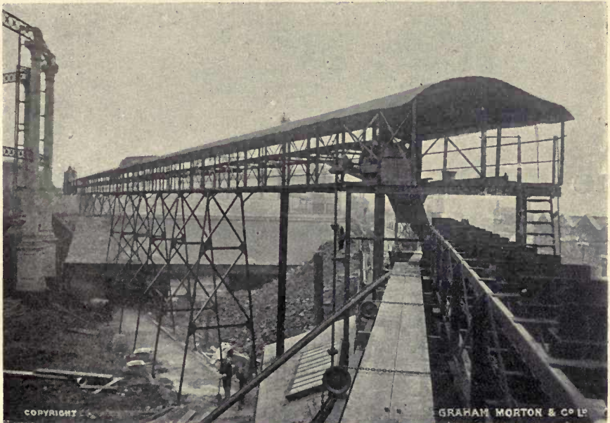
VIEW SHOWING A 35-TON CONVEYING AND STORAGE PLANT.
