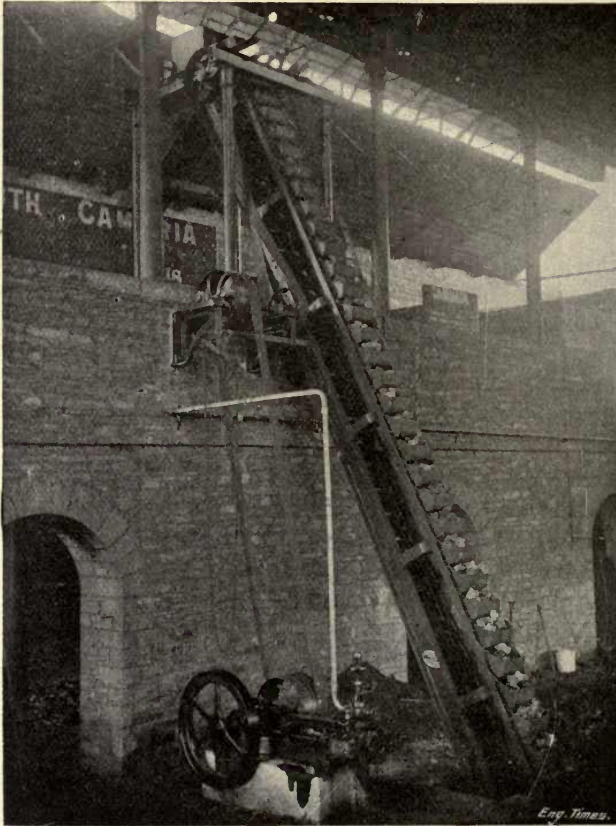
FIG. 38.—COKE ELEVATOR FILLING RAILWAY WAGGONS.
