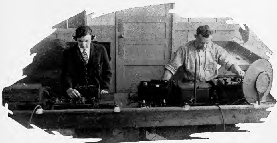
Testing "B" Eliminators in the General Radio Laboratories.
