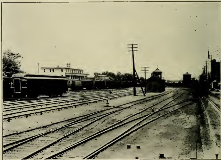
THE YARDMASTER'S OFFICE — IN AN ABANDONED SWITCH-TOWER
