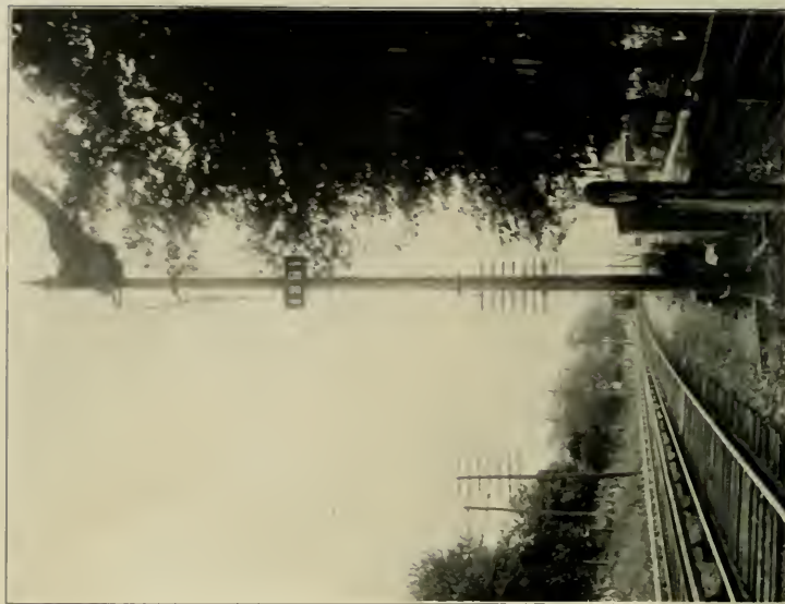
THE NEW YORK CENTRAL IS ADOPTING THE NEW FORM OF "UPPER QUADRANT" SIGNAL
