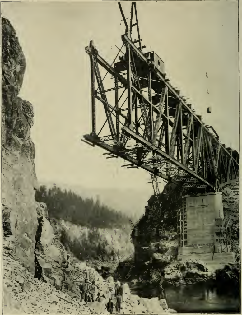
BUILDING THE WONDERFUL BRIDGE OF THE IDAHO & WASHINGTON NORTHERN OVER THE PEND OREILLE RIVER, WASHINGTON
