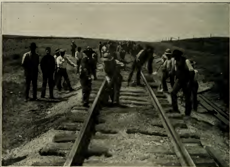
THE FINISHING TOUCHES TO THE TRACK
