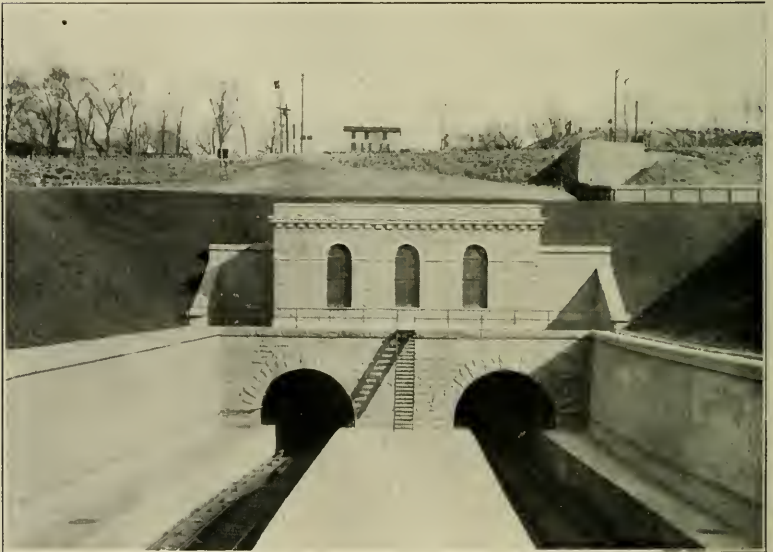
THE HACKENSACK PORTALS OF THE PENNSYLVANIA'S GREAT TUNNELS UNDER NEW YORK CITY
