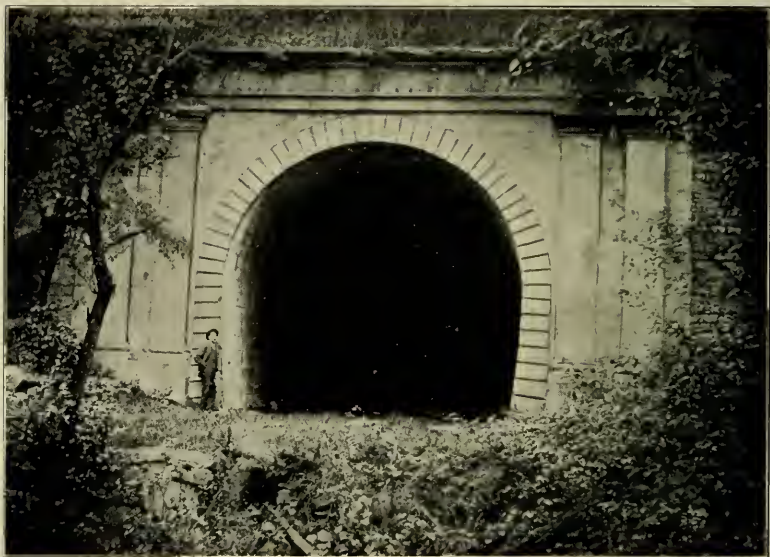
PORTAL OF THE ABANDONED TUNNEL OF THE ALLEGHANY PORTAGE RAILROAD NEAR JOHNSTOWN, PA., THE FIRST RAILROAD TUNNEL IN THE UNITED STATES
