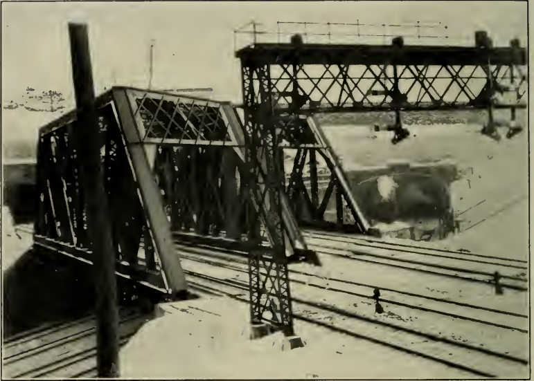
THE BUSIEST TUNNEL POINT IN THE WORLD — AT THE WEST PORTALS OF THE BERGEN TUNNELS, SIX ERIE TRACKS BELOW, FOUR LACKAWANNA ABOVE
