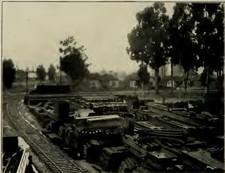
THE BRIDGE-BUILDER LAYS OUT AN ASSEMBLY-YARD FOR GATHERING TOGETHER THE DIFFERENT PARTS OF HIS NEW CONSTRUCTION
