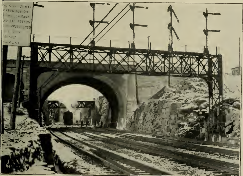
ENTRANCE TO THE GREAT FOUR-TRACK OPEN CUT WHICH THE ERIE HAS BUILT FOR THE COMMUTER'S COMFORT AT JERSEY CITY
