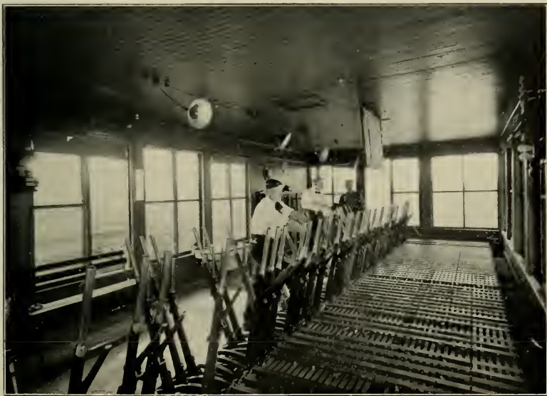
THE RESPONSIBLE MEN WHO STAND AT THE SWITCH-TOWER OF A MODERN TERMINAL: A LARGE TOWER OF THE "MANUAL" TYPE
