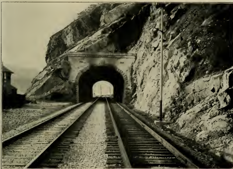
LINE REVISION ON THE NEW YORK CENTRAL—TUNNELLING THROUGH THE BASES OF THESE JUTTING PEAKS ALONG THE HUDSON RIVER DOES AWAY WITH SHARP AND DANGEROUS CURVES
