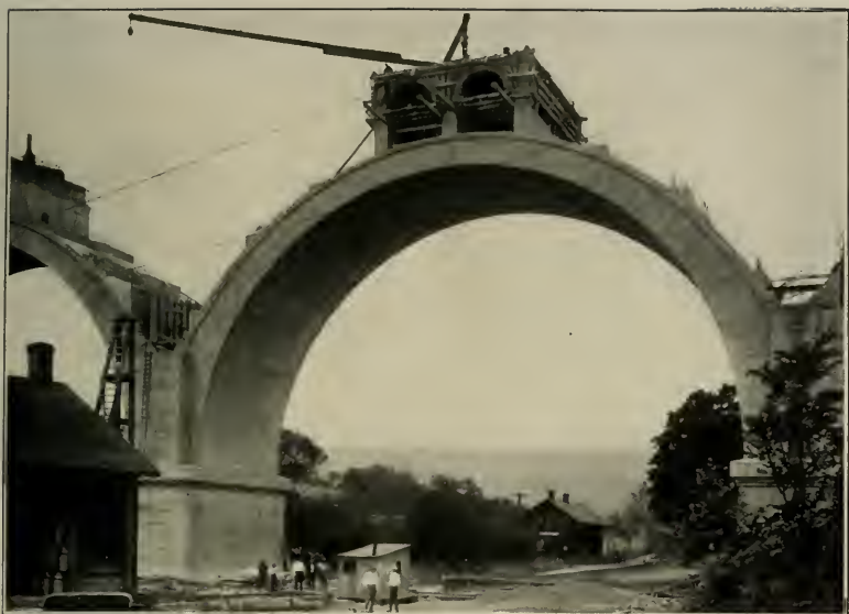
CONCRETE AFFORDS WONDERFUL OPPORTUNITIES FOR THE BRIDGE-BUILDERS
