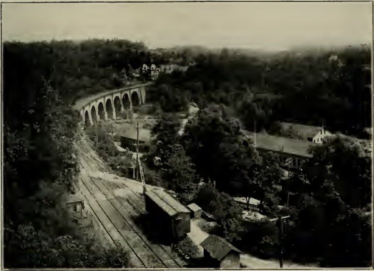
THE FAMOUS THOMAS VIADUCT, ON THE BALTIMORE & OHIO AT RELAY, MD., BUILT BY B. H. LATROBE IN 1835, AND STILL IN USE
