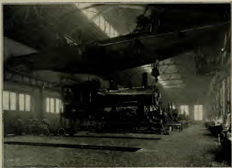
INSIDE THE WEST ALBANY SHOPS OF THE NEW YORK CENTRAL: PICKING UP A LOCOMOTIVE WITH THE TRAVELLING CRANE
