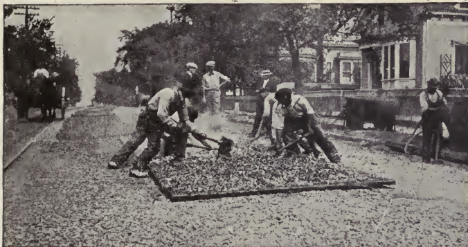
Fig. 66. Hand Method of Mixing Stone and Binder Courtesy of Barrett Manufacturing Company, New York City
