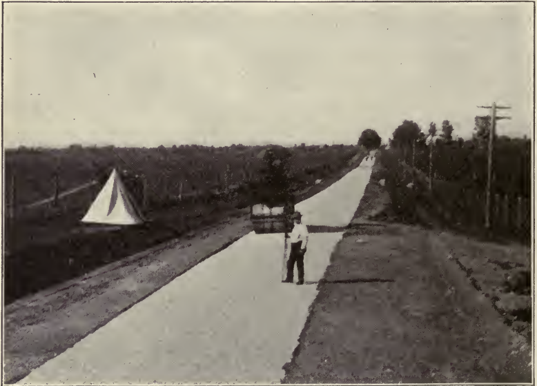
Fig. 63. Compacting Broken Stone by Steam Roller Courtesy of United States Department of Agriculture
