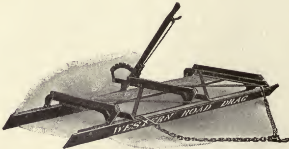
Fig. 60. Steel Road Drag
