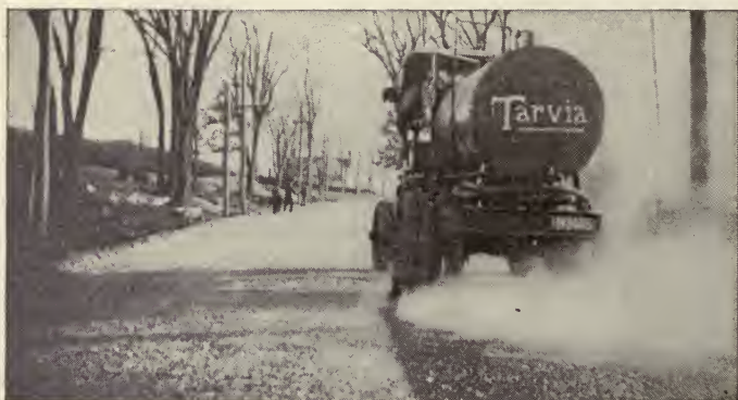
Fig. 69. Spraying Seal Coat by Auto Truck, One-Half Gallon to the Yard Courtesy of Barrett Manufacturing Company, New York City
