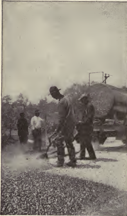
Fig. 65. Spreading Bituminous Binder by Pressure Nozzle, Penetration Method Courtesy of Barrett Manufacturing Company, New York City
