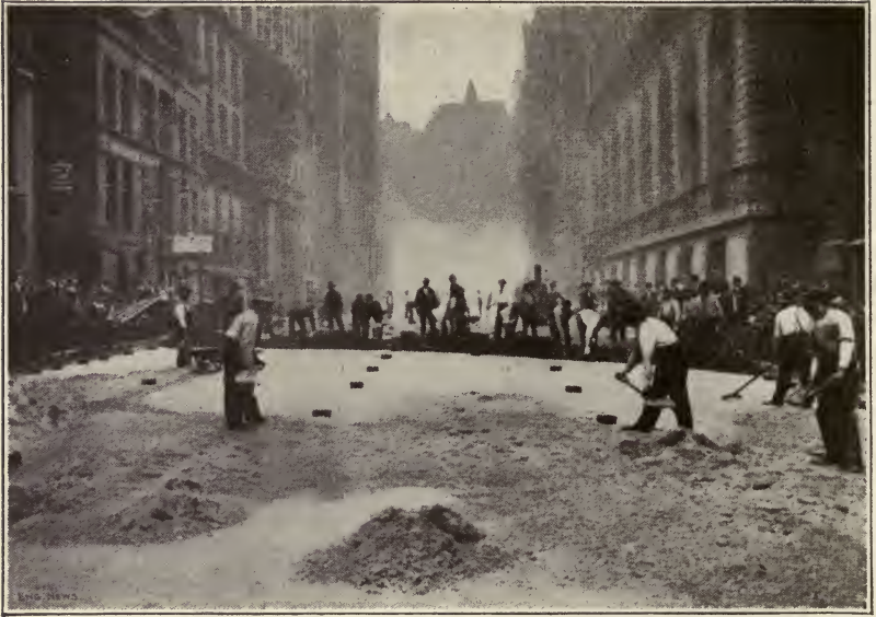
Fig. 92. Spreading Sand Foundation for Wood Blocks in LaSalle Street, Chicago Courtesy of Engineering News, New York City
