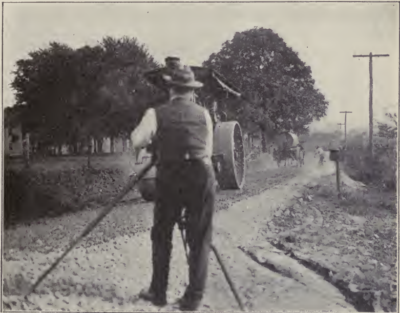
Fig. 64. Rolling and Sprinkling Second Course of Macadam Road to Complete Binding Process
