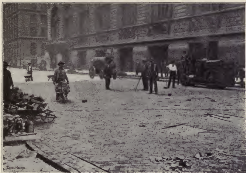
Fig. 94. Wood-Block Pavement Being Hammered and Rolled, Preparatory to Putting in Filler Courtesy of Engineering News, New York City
