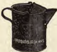
Fig. 100. Pouring Pots Used with Asphalt Pavements Courtesy of Barber Asphalt Paving Company
