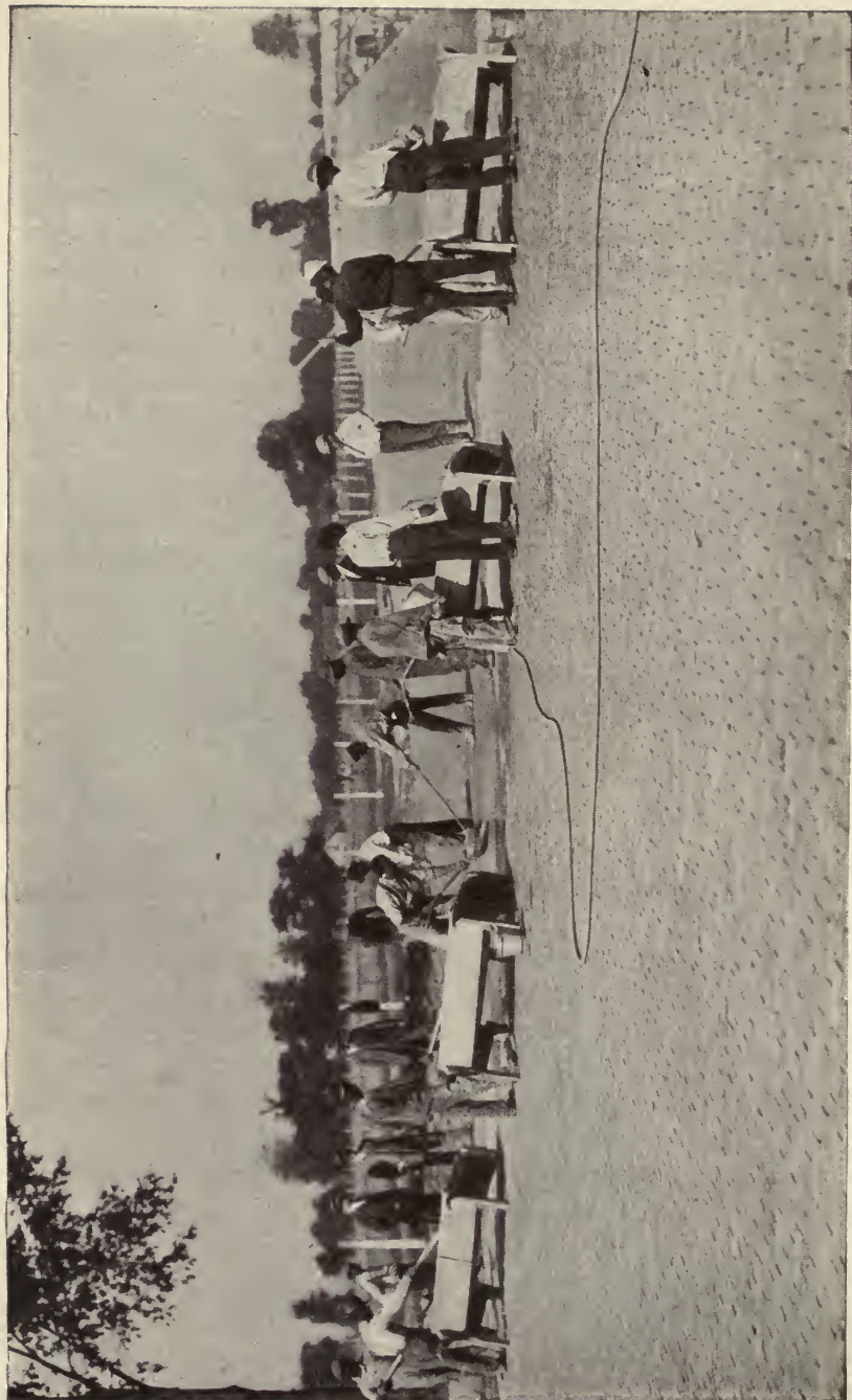
Fig. 87. Street Laying Gang Applying Filler to Brick Pavement Courtesy of National Paving Brick Manufacturers Association, Cleveland, Ohio
