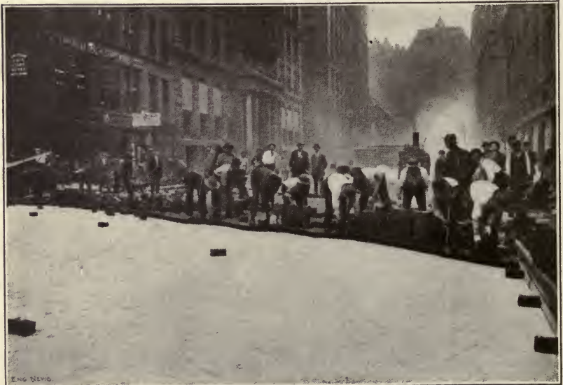
Fig. 93. Laying Wood Blocks in LaSalle Street, Chicago Courtesy of Engineering News, New York City
