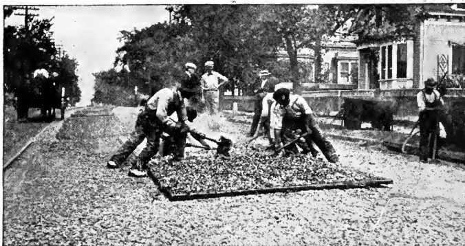
Fig. 66. Hand Method of Mixing Stone and Binder Courtesy of Barrett Manufacturing Company, New York City
