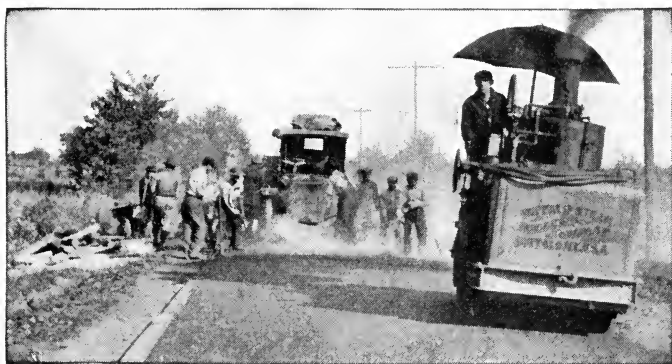
Fig. 68. Rolling Bituminous Macadam Road Surface Courtesy of Barrett Manufacturing Company, New York City
