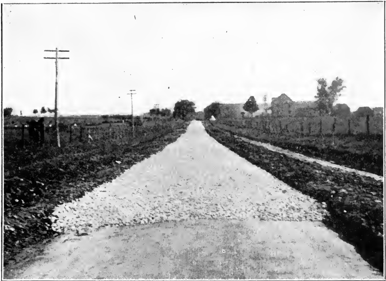
Fig. 62. View Showing Spreading of Lower Course of Macadam Road Courtesy of United States Department of Agriculture
