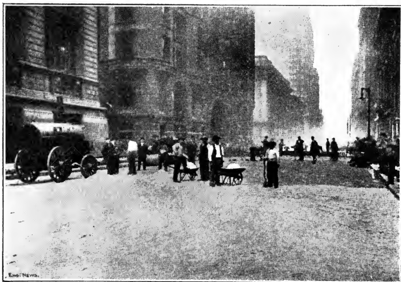
Fig. 95. Spreading Sand Filler on Wood-Block Pavement Courtesy of Engineering News, New York City
