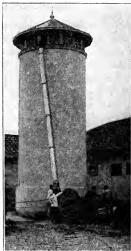
Fig. 27.— Cement Silo and No. 17 Ohio Cutter at Experiment Station, Sao Paulo, Brazil.
