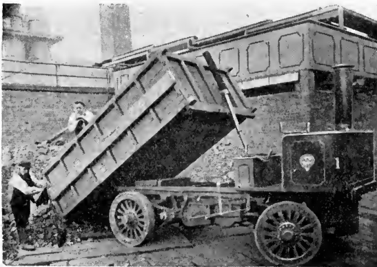
Fig. 70. Telescopic-Screw Tipping Gear.
