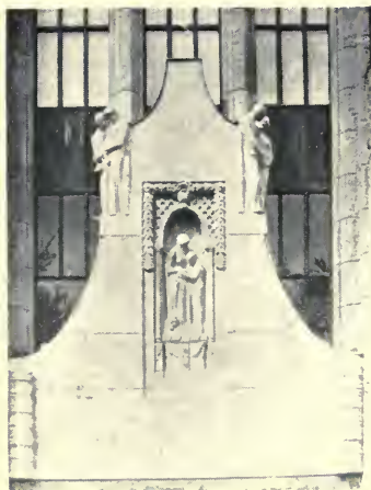
175. METZNER: DETAIL OF HAUS TIETZ
