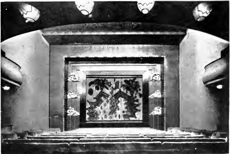
209. SIEBURG: PROSCENIUM OF MARBLE HOUSE THEATER
