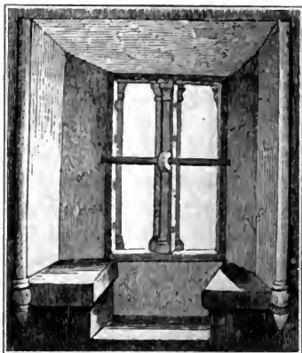
INTERIOR VIEW OF THE UPPER WINDOW SHOWN IN MELICHOPE MANOR HOUSE. This view shows the depth of the wall,—into which, indeed, the stairway is cut.
