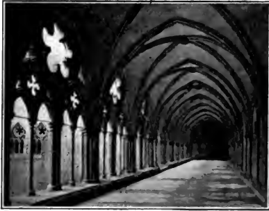
SALISBURY CLOISTERS. Note the intersecting ribs of the vaulted ceiling (§ 285).
